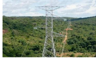
Transmission and distribution of electricity
