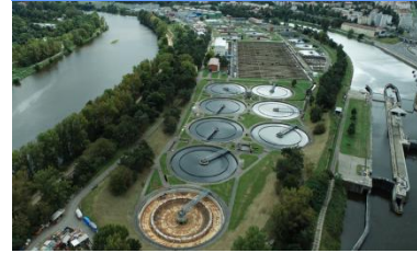
Water treatment plants and networks
