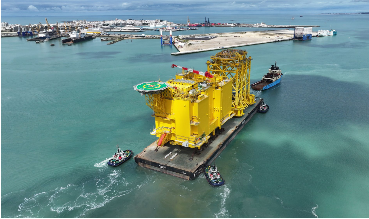
BorWin5, the HVDC converter platform built by Cobra IS and Siemens Energy for TenneT has been installed in Germany
