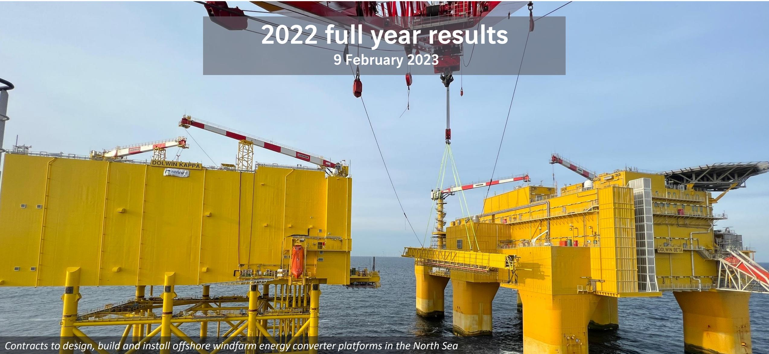
*Contracts to design, build and install offshore windfarm energy converter platforms in the North Sea*
