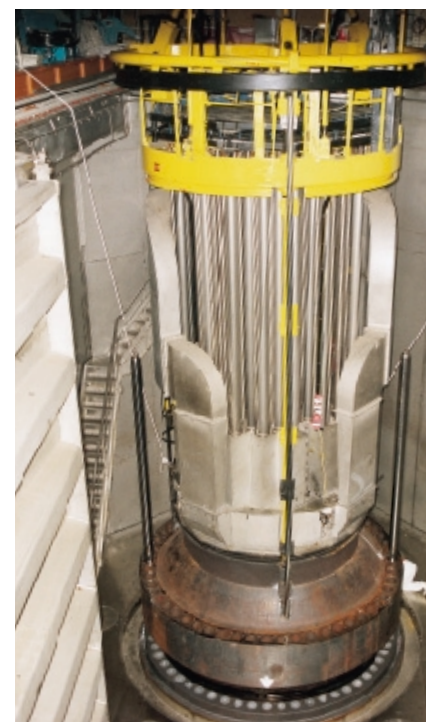
Nuclear reactor vessel opening and closing operation.
