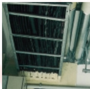
Fire protection coating of electrical cable conduits.
