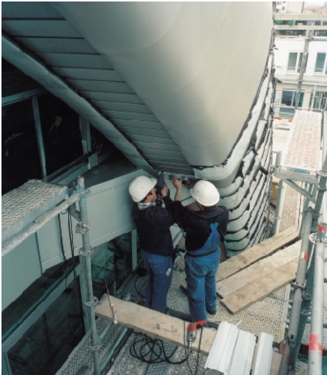
G+H MONTAGE produced 4,000 tailor-made pieces of stainless steel to cover the "Tattoo" roof in Berlin, Germany.
