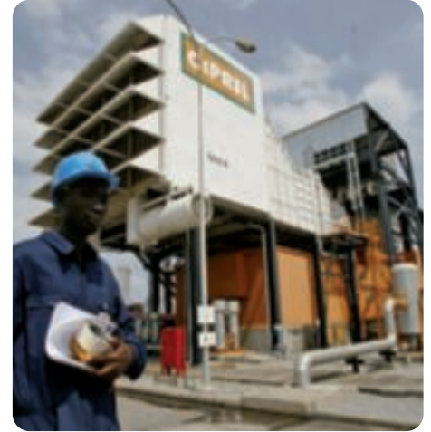
Extension of a thermal power plant in Abidjan, Ivory Coast.
