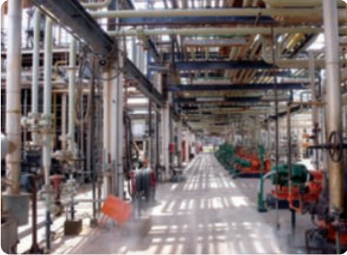
Revamping electrical networks at the Arzew refinery in Algeria.
