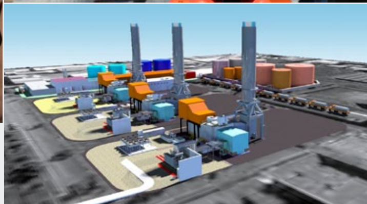
3D model of the planned Kenitra power station, comprising three turbines and stacks, fuel oil and water storage and treatment installations, and 2,000 square metres of utility buildings.
