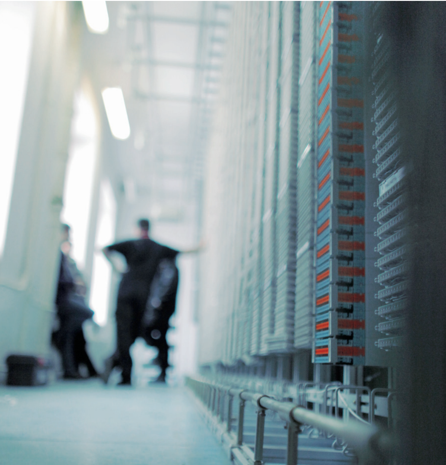
ORANGE POLSKA TELEPHONE SWITCHBOARD IN OPOLE (POLAND) Graniou Atem has been working for several years with Orange Polska to develop new-generation networks in Poland.
