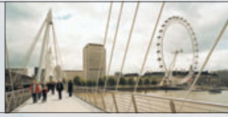
▶ Hungerford Footbridges, London
