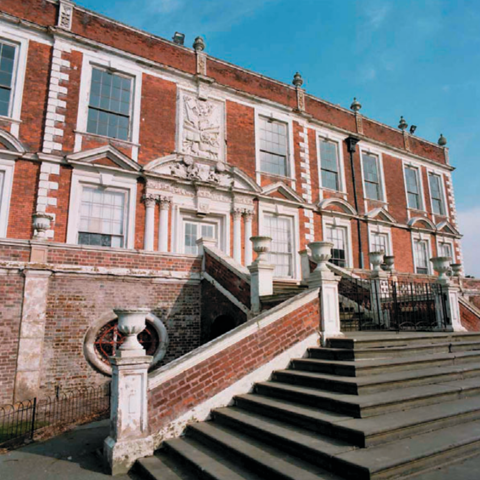
▲ Croxteth Park Liverpool Vinci Services Ltd Maintenance of Liverpool's Public Buildings
