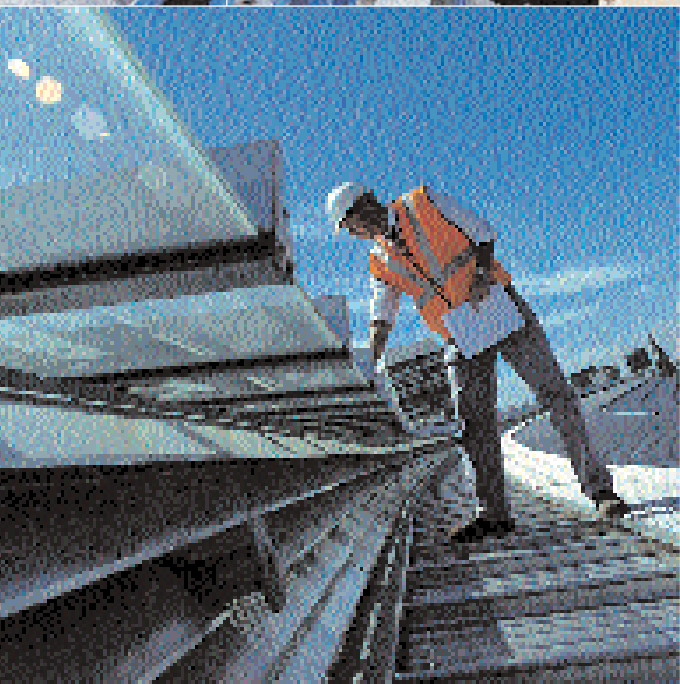
◀ Liverpool Lime Street Station re-roofing
