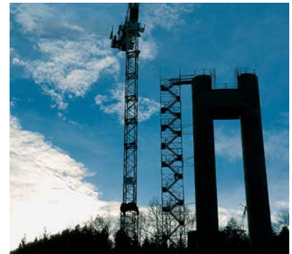
Design and construction of the 900 metre long Monestier viaduct on the A51 motorway (GTM GCS).
