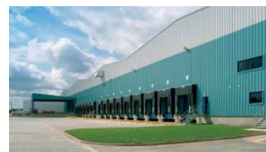
New 22,000 square metre distribution centre for L'Oréal in Manchester, United Kingdom (VINCI PLC).
