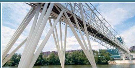
Footbridge at the Science Museum in Valladolid, Spain. The metal structure has longitudinal and transverse prestressing.
