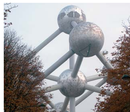
Nizet is renovating electrical systems and outdoor lighting at the Atomium, the famous monument in Brussels, which is more than 100 metres high.
