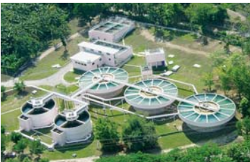
Water treatment plant built as part of the Great River project in Jamaica (VINCI Construction Filiales Internationales/Sogea Construction).
