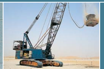
Dynamic compacting of a 3.5 million square metre pavement support in Abu Dhabi (Ménard Soltraitement).
