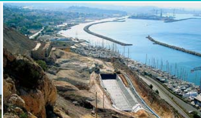
Rehabilitation of former industrial facilities at the port of Estaque in Marseille (GTM Terrassement).
