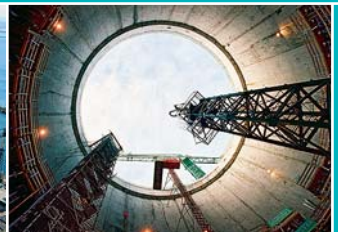
Construction of a 75 metre deep underground missile facility in Biscarosse, south-west France.
