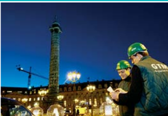
Rehabilitation of a 30,000 square metre complex in the Place Vendôme in Paris (GTM Bâtiment/Dumez IDF).
