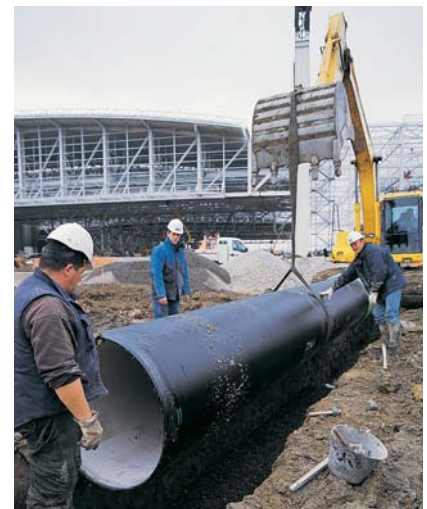
Installation of underground networks at the Aéroconstellation development zone in Toulouse Blagnac (Sogea Sud-Ouest).
