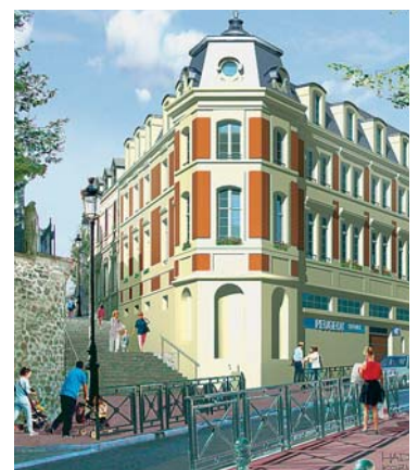
Municipal administration building in Le Plessis Robinson, near Paris, built under a long-term lease by Sogea Construction.
