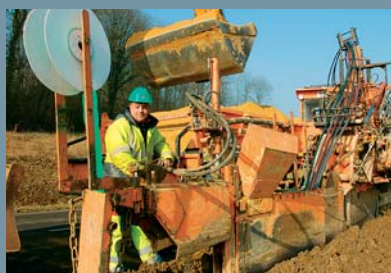
Mechanised laying of optical fibre cables. VINCI Construction installs and manages networks under public service outsourcing contracts.
