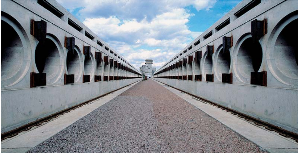
At the site of the Chernobyl nuclear power station, VINCI Construction Grands Projets handed over the civil engineering work on the conditioning plant and the storage unit for the spent fuel from the units that have been shut down.
