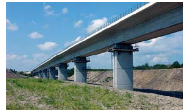
Construction of an 800 metre bridge near Chomutov in the Czech Republic (SMP).
