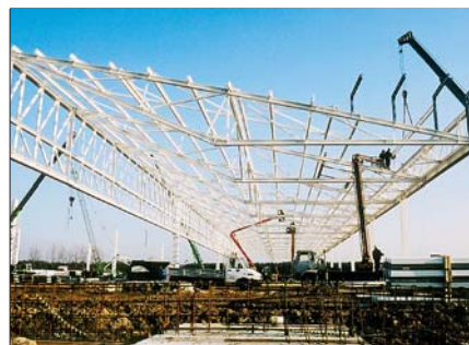
New plant for equipment manufacturer Valeo in Chrzanow, Poland (Warbud).
