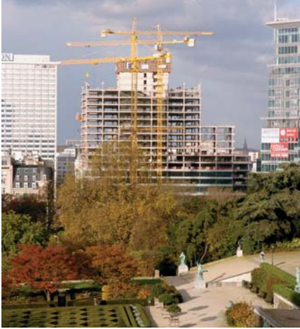
Rogier tower (36 storeys, 125,000 square metres), built by CFE for Dexia in Brussels.
