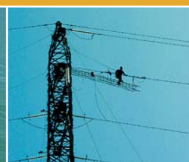
Engema performs maintenance on the Beerst-Koksidge high voltage line.
