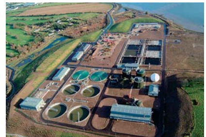
Civil engineering at the wastewater treatment plant in Cork, Ireland (16 tanks and five buildings), handed over in 2004.
