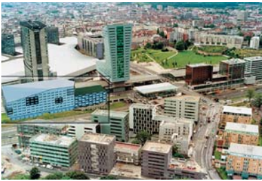
Axe-Europe project (23,000 square metres of office space, 16,000 square metres of car parks) built by Sogea Construction for Elige in Lille.
