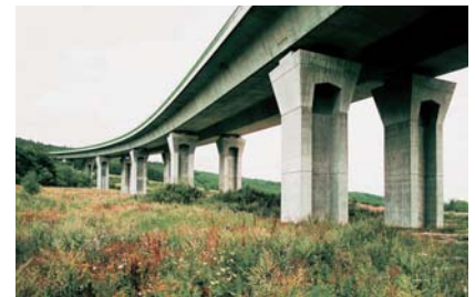
800 metre long segmental bridge built by SMP near Chomutov in the Czech Republic.
