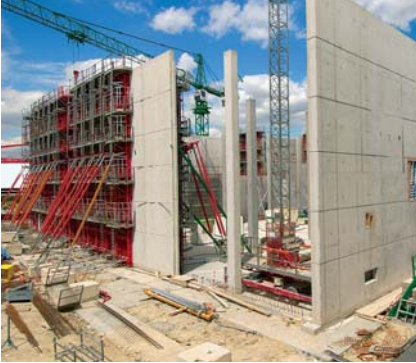
Valenton sludge treatment facility (with a capacity of 600,000 cubic metres per day) in the Paris region (Sogea Construction/GTM Construction).
