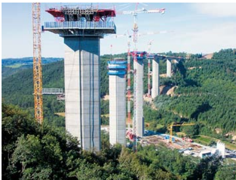
La Sioule viaduct (990 metres long, with a 192 metre central span) built by Sogea Construction on the A89 motorway.
