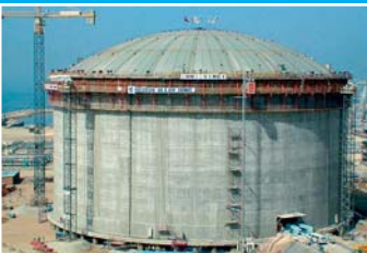
One of the two 140,000 cubic metre liquefied natural gas tanks in Idku, Egypt.
