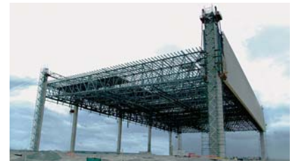
A 3,000 tonne truss covering an airport hangar in Brisbane, Australia was raised 25 metres.
