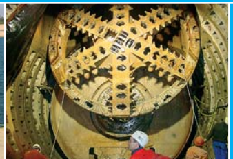
The Lefortovo road tunnel in Moscow, bored by a mud-pressure tunnel-boring machine.
