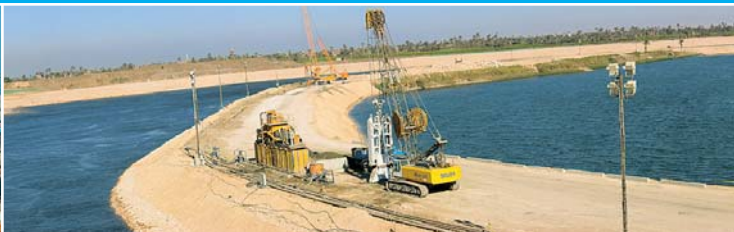
The Naga Hammadi dam, 150 km north of Luxor, designed to control the flow of the Nile and provide irrigation and power generation, is to be completed in 2008.
