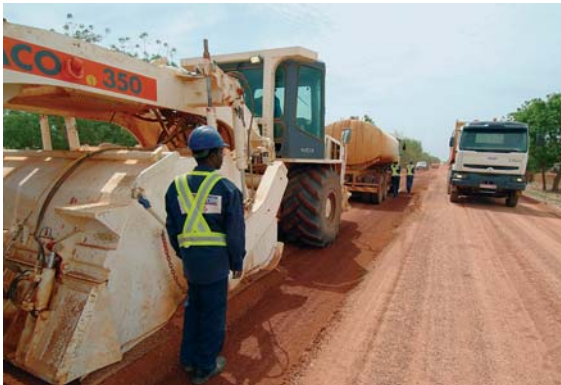
Redevelopment of National Highway 1 in Niger (Guidam Roundji-Maradi-Tchadoua section); following this work, Sogea-Satom will be restoring the quarries and re-planting vegetation.
