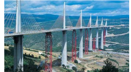
In just 55 days, Freyssinet installed the 154 stay cables (1,500 tonnes) of the Millau viaduct, built by the Eiffage Group in France.
