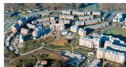
The Jardins de la Jette in Brussels, an office, residential and retail complex developed and built by CFE.
