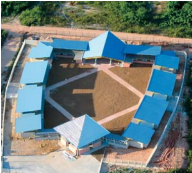
Construction of a primary school in the shape of a leathery turtle in Saint Laurent du Maroni, French Guiana (Nofrayane).
