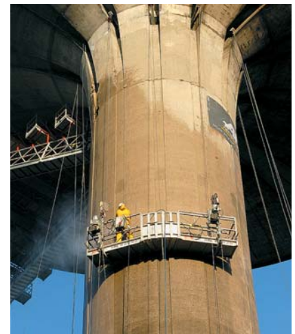
Rehabilitation of the water tower at Roissy-Charles de Gaulle Airport in the Paris region.
