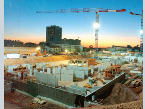
Toulon military hospital, one of the largest hospital complexes currently under construction in France (Sogea Construction).
