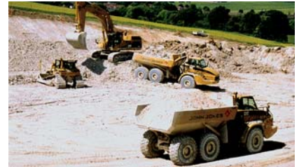
John Jones Excavation is carrying out the earthworks on the Baldock bypass in Hertfordshire.
