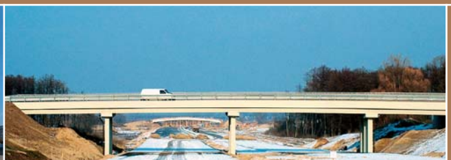
In Hungary, Hídépítő is building 15 bridges and three viaducts on a 20 km section of the M7 motorway (Balatonszarszo-Ordascehi).
