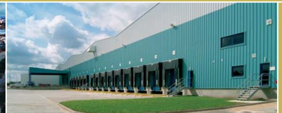
Design and construction of the new L'Oreal distribution centre in Manchester (22,000 square metre warehouse and two buildings with floor areas of 1,650 and 1,900 square metres respectively).
