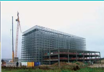
Construction of two 100,000 cubic metre warehouses for Miko in Saint Dizier (GTM GCS Agence Lorraine).
