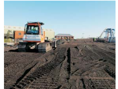
On the Newport bypass worksite in the United Kingdom, 42% of the backfill used in earthmoving was ballast recovered from railway renovation projects.
