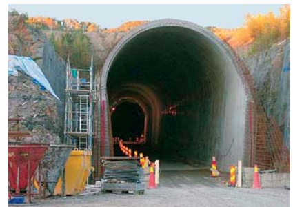
5.6 km Hallandsas rail tunnel on the high-speed line between Gothenburg and Malmö in Sweden.
