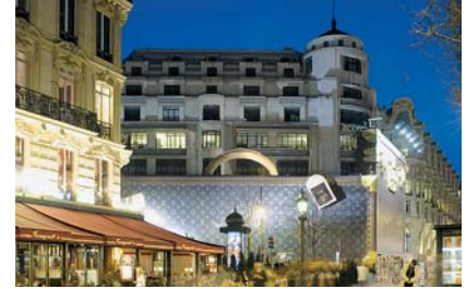
Structural renovation of the Louis Vuitton showroom on the Champs Elysées in Paris (Entreprise Petit).
