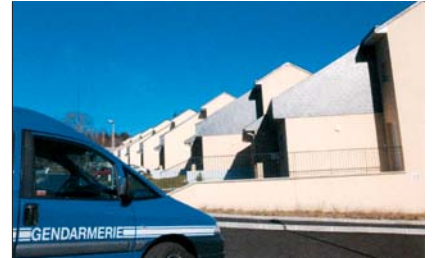
Sogea and GTM put together several gendarme station projects under long-term leases.
