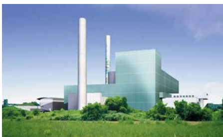
VINCI Construction builds household waste incineration facilities (shown here, the facility in Carrières sur Seine) and modernises their flue gas scrubbing equipment.
