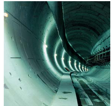
Boring of the Toulouse metro and civil engineering for metro stations (GTM Construction/Sogea Construction).
