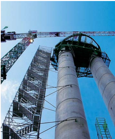
Monestier de Clermont viaduct (900 metres long) on the A51 motorway in south-eastern France (GTM Construction).
