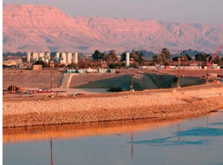
In Egypt, construction of the Naga Hammadi dam by VINCI Construction Grands Projets required a diversion of the Nile for the second time in history.
