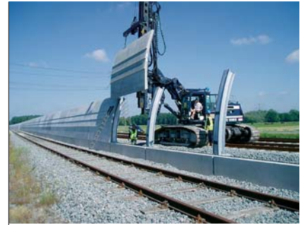
Installation of sound barriers over a 90 km stretch of the Betuweroute in the Netherlands (CFE).
