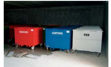
VINCI Construction is extending selective sorting and collection of waste to all its worksites.
