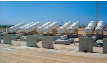
Al Gardabiya Assdada pumping stations in Libya (VINCI Construction Grands Projets).
