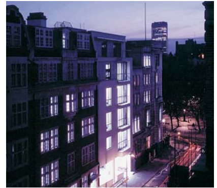
Construction at the new Great Ormond Street Hospital for Children in London.
