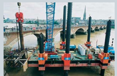
Consolidation of the piles for the Pierre bridge in Bordeaux (Sogea Construction).
