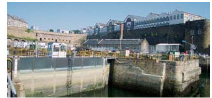
Renovation of two dry docks at the Brest shipyard, requiring 18,000 cubic metres of concrete (GTM GCS).
