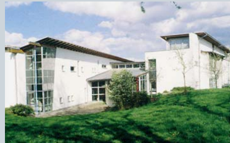
As part of a 15 year contract covering 43 schools, SKE will be spending €80 million on renovation work.
