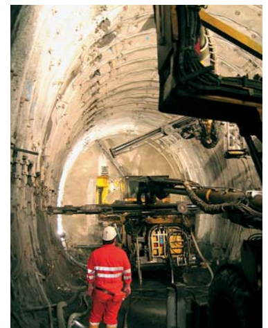
Mitholz rail tunnel in Switzerland (VINCI Construction Grands Projets).
