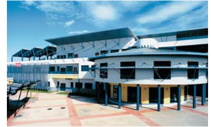
Construction of the Saint-André school on Reunion (SBTPC).
