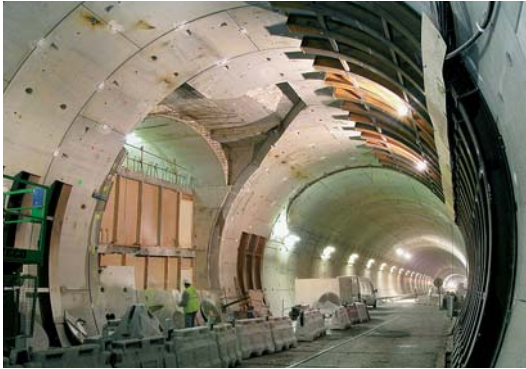
First (4.5 km) section of the tunnel completing the A86 West motorway in the Paris region (VINCI Construction Grands Projets/GTM Construction/Sogea Construction).
