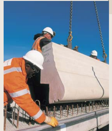
In 2003, VINCI Construction Grands Projets launched an accident prevention - safety challenge designed to raise awareness among all its teams (seen here on the CTRL construction site in the UK).
