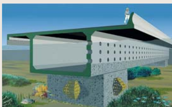
The Grand Prize at the 2003 VINCI Innovation awards went to the green breakwater, a new type of underwater concrete structure which promotes natural renewal of water and rapid colonisation by flora and fauna.
