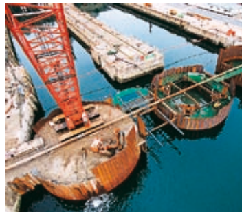
Refurbishment of the drydocks (2 and 3) in the Brest shipyards (GTM Bâtiment).
