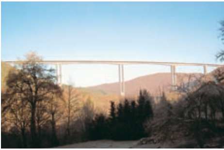
Sioule Viaduct (990 metres long; 192 metre central span): a major structure on the last section of the A89 motorway linking Clermont Ferrand and Bordeaux.
