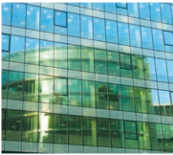
Palatin II and III Buildings in La Défense, handed over in 2005 (GTM Bâtiment, Petit).
