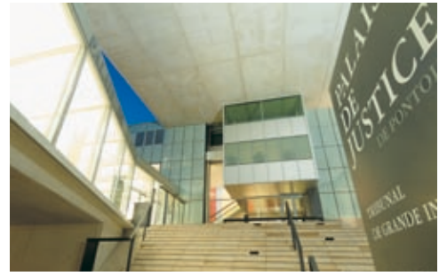
The new Pontoise courthouse (11,800 sq. metres, 270 parking spaces) built by GTM Bâtiment on a general contracting basis and handed over in 2005.
