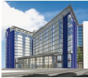
Construction of a 13-storey, 284-room hotel in Manchester for City Inn Ltd.
