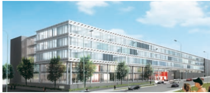
New building for RTL, one of the many construction projects currently being carried out by CFE in Brussels.
