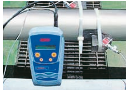
Fluidis-WMI's water treatment design-build offering complements its water distribution network audit and repair capabilities.
