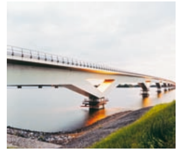
Moerdijk Bridge along the HSL4 rail line in Dordrecht, Netherlands.
