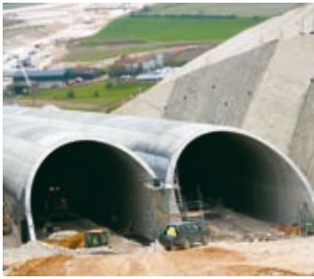
6.5 km Baldock bypass in Hertfordshire, comprising a 250 metre cut-and-cover tunnel.
