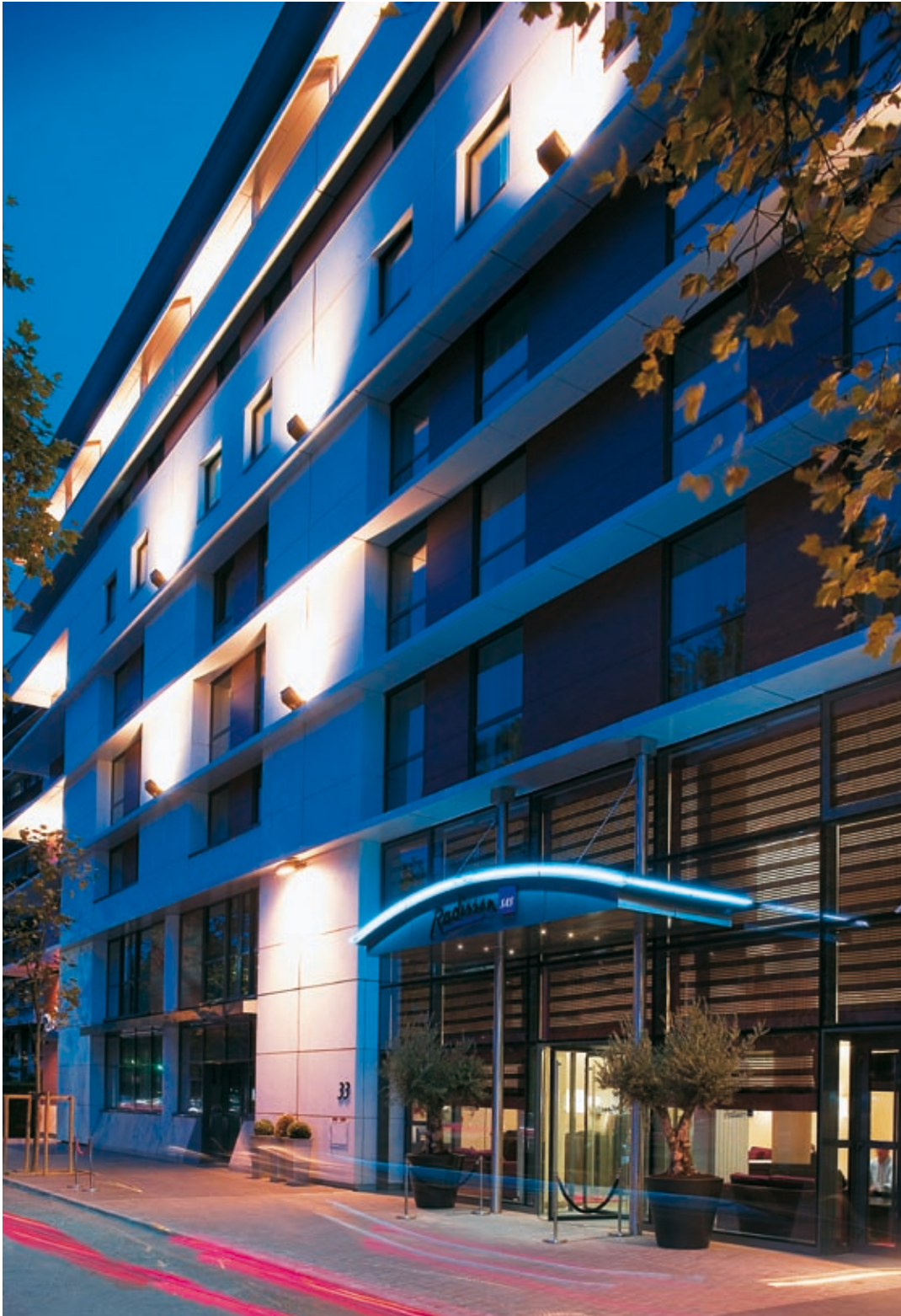
Radisson Hotel in Boulogne Billancourt (170 rooms) in the greater Paris region, handed over in 2005 (Campenon Bernard Construction).
