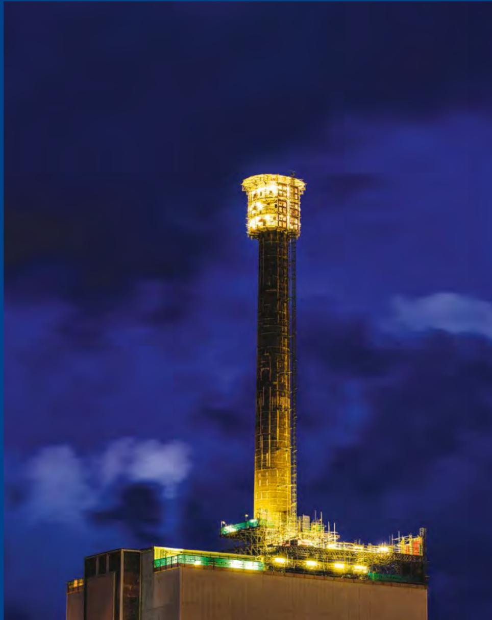
© Self-Climbing Palform pictured nearing the final descent of the FGRP Stack demolition
