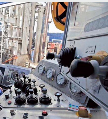
01. France – Geothermal drilling in Coulommiers.
