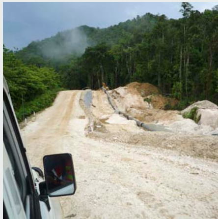
Papua New Guinea – Reinstatement following pipeline installation. PNG project.
