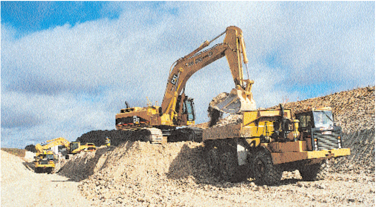
The Civil Engineering Division of Norwest Holst Construction is currently undertaking a joint venture contract to build the mid-Kent section of the Channel Tunnel Rail Link. Specialist subsidiary, John Jones (Excavation) Limited, is undertaking two contracts for bulk earthworks on two sections of the high speed rail link.
