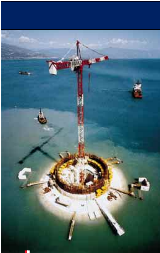
In 2004, the 2,883 meter long Rion-Antirion Bridge will cross the Gulf of Corinth to link the Peloponnese with western Greece. The main span is 2,280 meters in length and will rest on four piers in the sea designated M1, M2, M3 and M4. These supports will be the largest ever constructed for a bridge.
