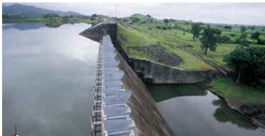
The Kakdiamba dam in India supplies drinking water to sixteen villages and irrigates 1,460 hectares. It has 55 Hydroplus fusegates (1 x 1.8 m) which increase the capacity of the reservoir by 22% and thus boost annual agricultural production by nearly 310 tons.
