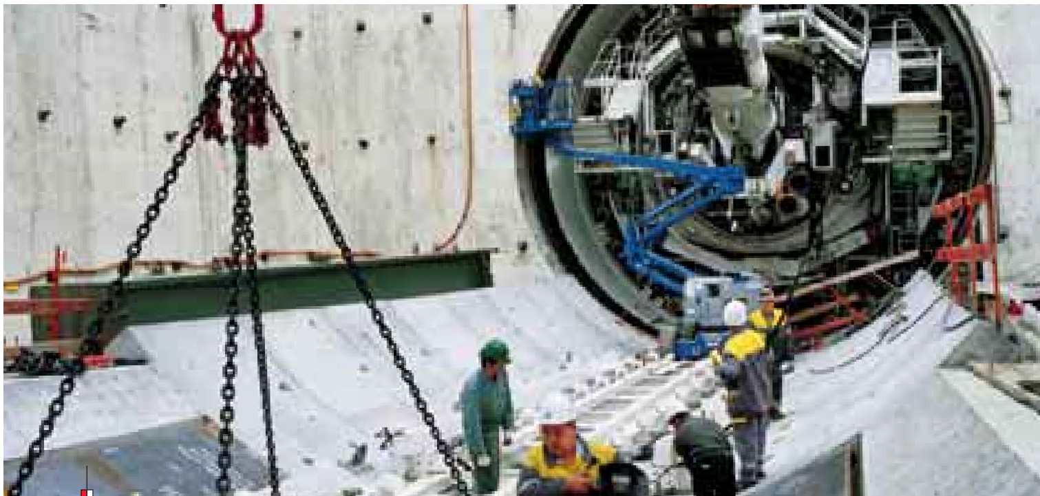
Work on the A86 West Motorway, interrupted for two years, resumed in February 2000 at the site of the Rueil interchange. Following assembly of the tunnelling machine, drilling of the Rueil-Malmaison / A 13 interchange began on 6 November 2000.
