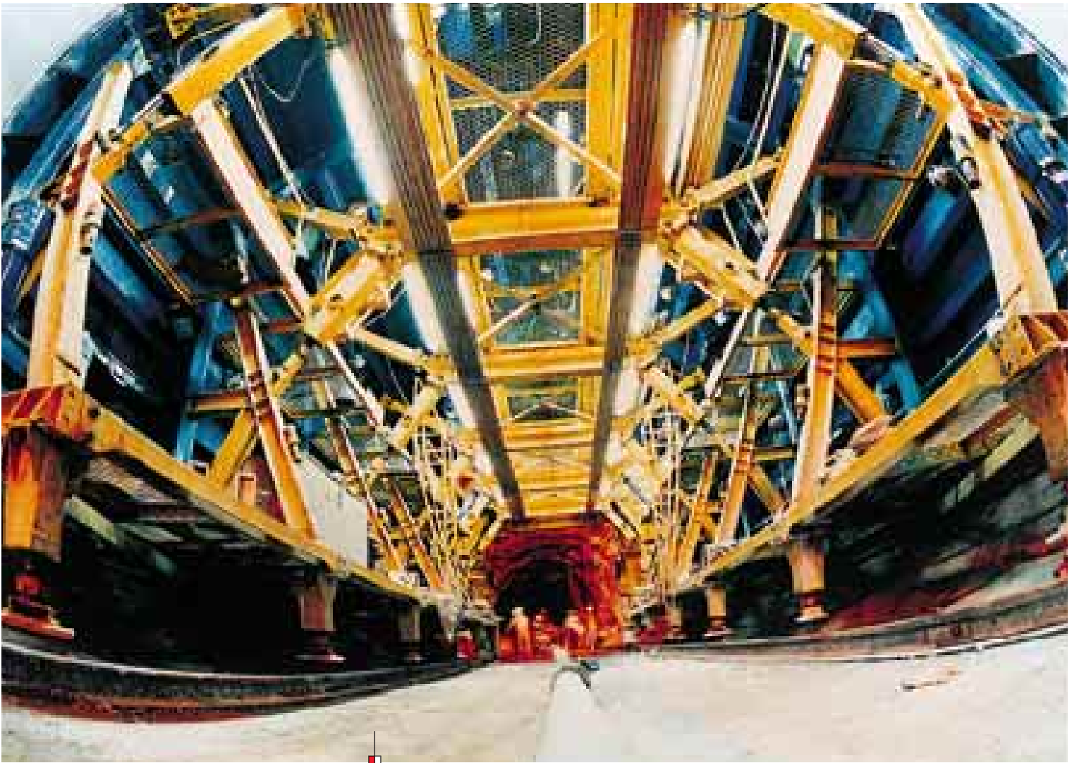
The design and build construction of works package 603 "Black Hill Tunnels" in Hong Kong required major technical innovations devised in partnership with the customer.
