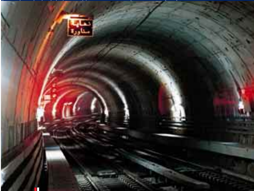
Handover of the second phase of line 2 of the Cairo Metro in Egypt took place in October 2000. It is a good illustration of successful organisation and preparation of a large design and build project on the international market.
