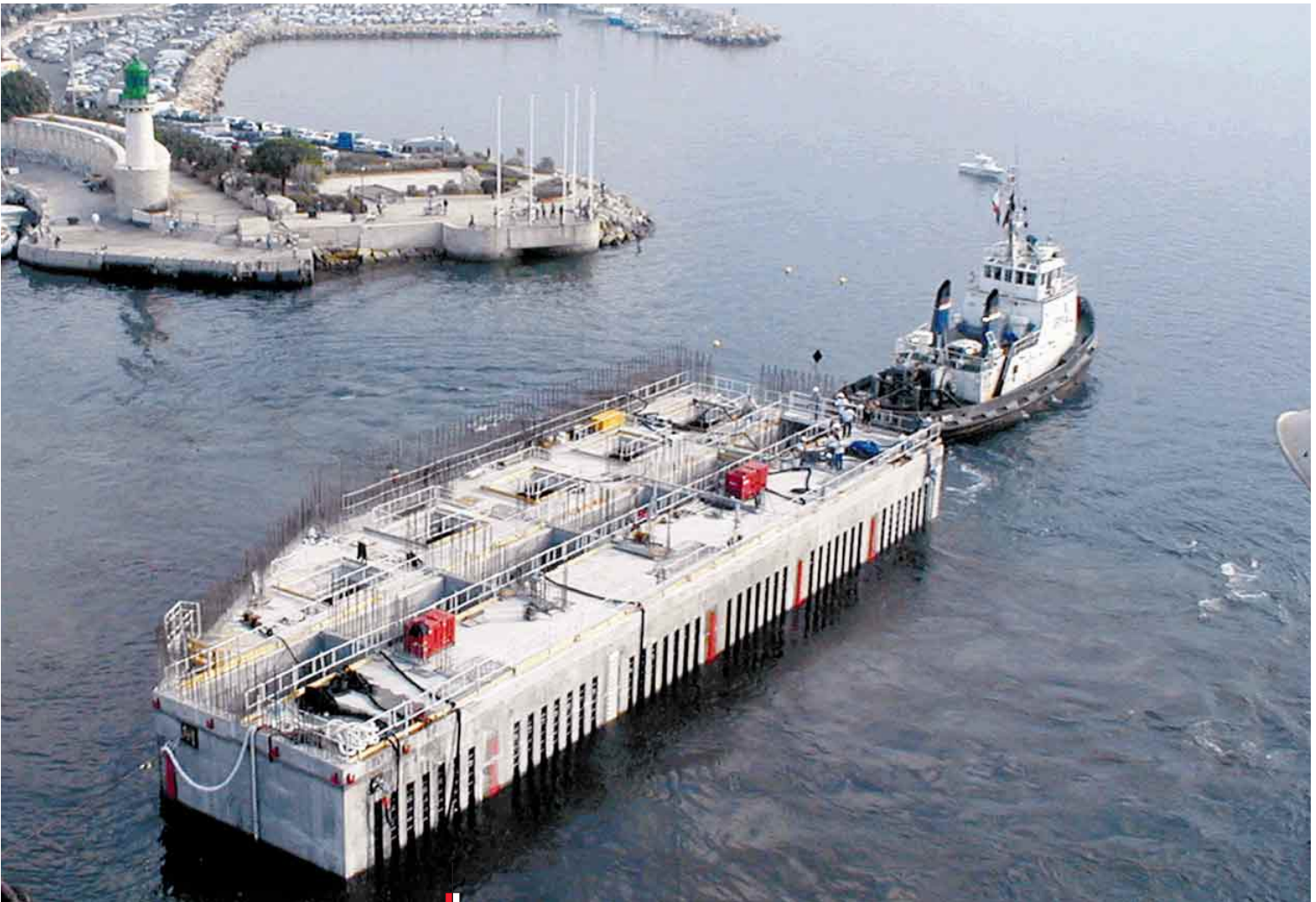
The design and construction of the 1-hectare quayage as part of the expansion of the Port of La Condamine in Monaco required the construction of 6 exceptional reinforced concrete caissons weighing between 15,000 and 35,000 tons.
