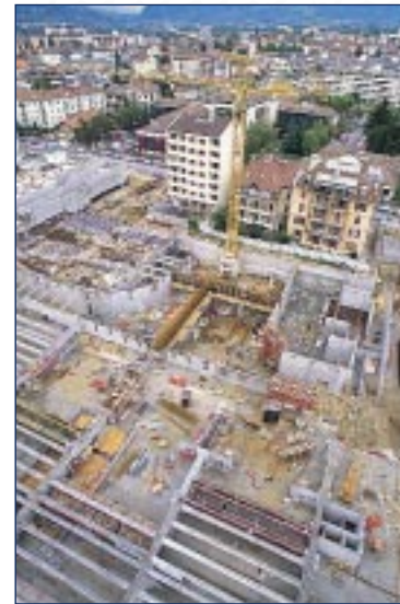
The ZAC Courier project in Annecy, involving the construction of a shopping centre, a cinema and a car park, requires the use of 54,000 cu. metres of concrete and more than 500 tonnes of steel.
