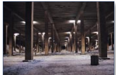
In addition to the purification plant itself, Campenon Saigon Builders is to refurbish the 10,000 cu. metre capacity underground drinking water reservoir no.3 of the Thu Duc water treatment plant.
