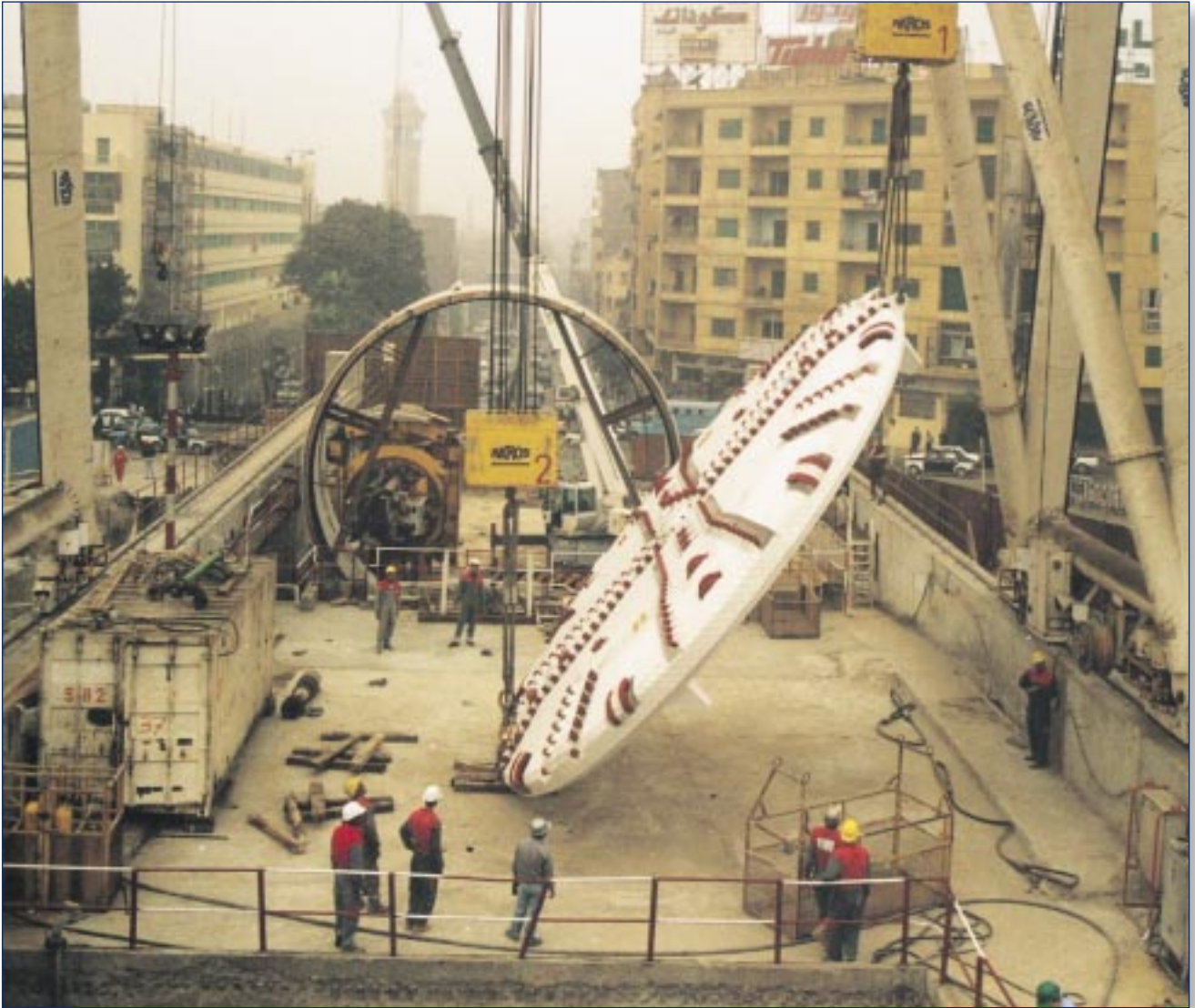
In Cairo, on the El Azhar road tunnel project, the technical challenge of building a 1,742 metre long underground crossing beneath the old town without damage to buildings overhead was met with complete success.
