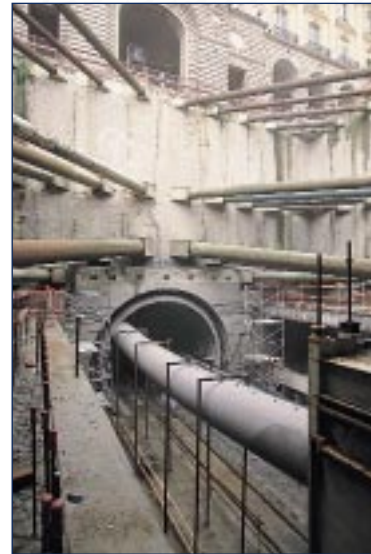
Terrain consolidation work on the route of the Rennes metro project made for a smooth crossing through the Vilaine river bed under the pont d'Orléans bridge.
