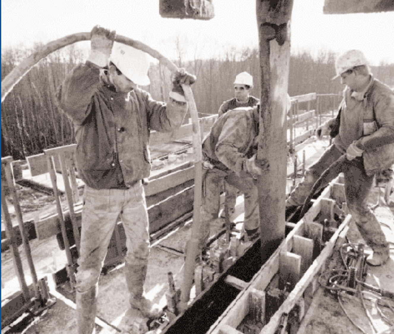
Construction of the drinking water plant at Méry-sur-Oise.
