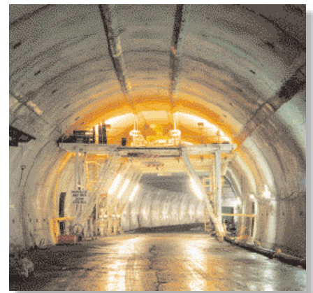
The Orelle tunnel, 3,680 metres in length, on the A43 Maurienne motorway.
