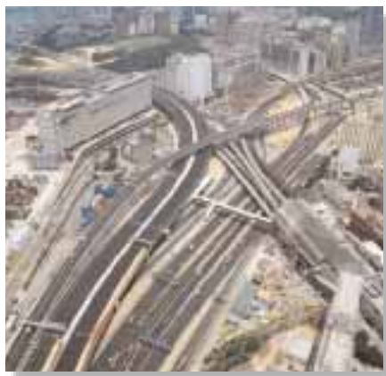
The 3.5 km-long Kwai Chung viaduct, completed in a record 45 months.
