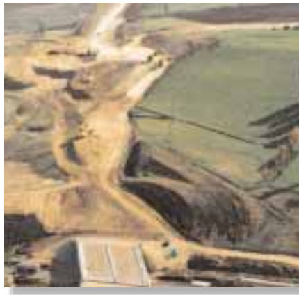
Earthworks on the A20 between Montauban and Caussade.
