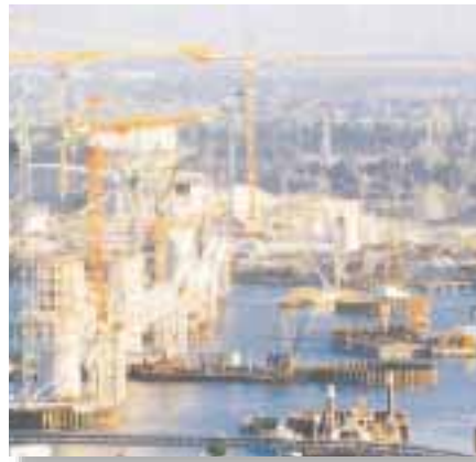
Construction of the bridge foundations for the Mornas and Mondragon viaducts north of the town of Orange, on the future Mediterranean TGV line.
