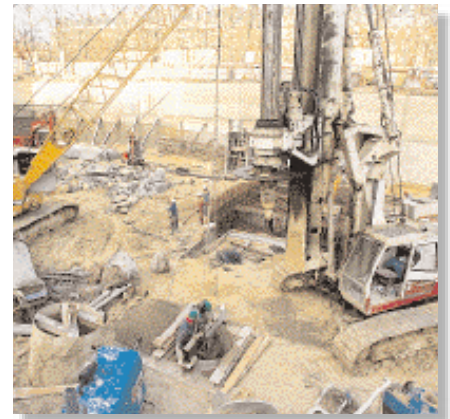
Botte BTP built the foundations for an office complex in the 14 th arrondissement of Paris.
