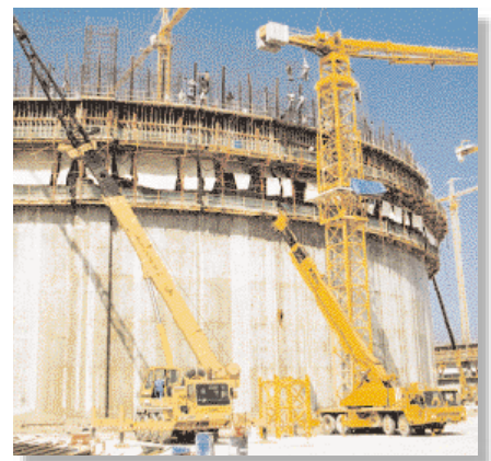
The outer shell of one of the three gas storage tanks in Qatar.
