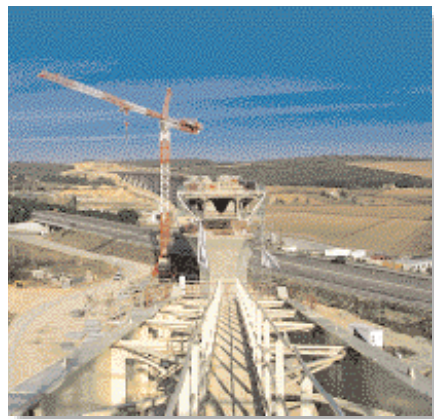
The piers of the incrementally launched north bridge of the Ventabren viaduct.
