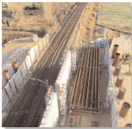
A bridge on the A77 motorway crossing over the Paris to Clermont-Ferrand railway line.
