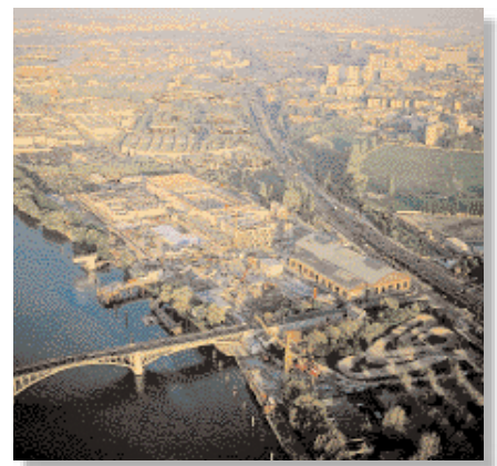
Initial testing of the partially below-ground purification plant at Colombes took place early in 1998.
