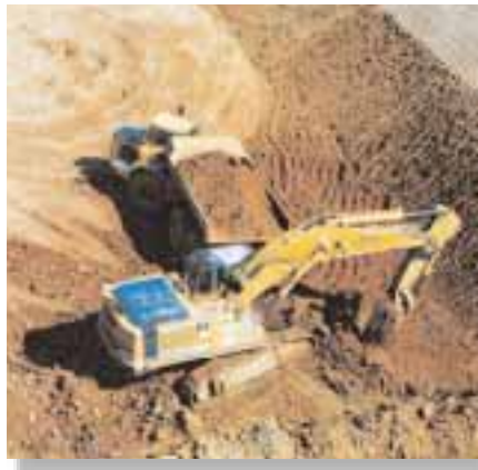
Earthworks on the future A29 motorway that will link Amiens and Le Havre.
