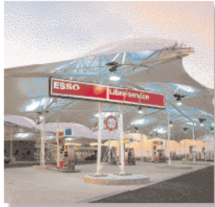
The futuristic Esso service station at Villeroy on the A19 motorway 130 kilometres south-east of Paris.
