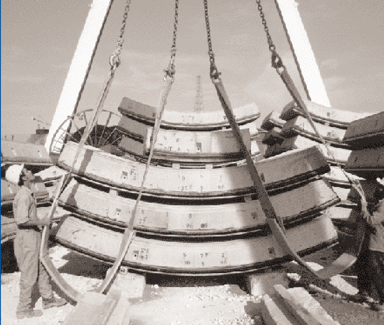
Boring of the tunnels for line 2 of the Cairo underground progressed strictly on schedule.
