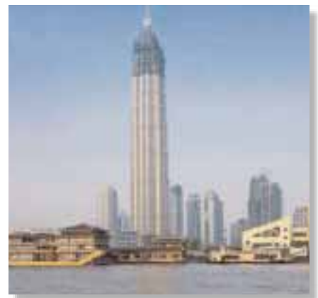
The Jin Mao tower in Shanghai : 420 m and 88 storeys high.
