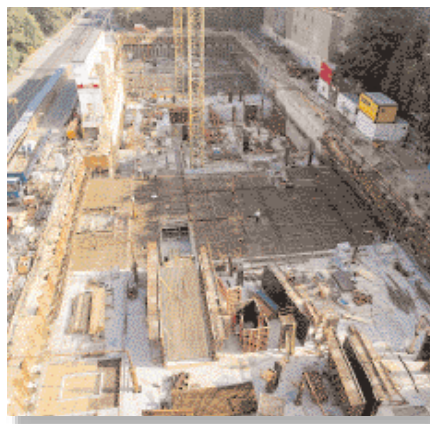
The Reinhardstrasse office complex project in central Berlin.
