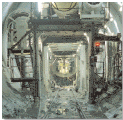
The Cachan-Charenton waste water collector was excavated with a tunnelling machine.
