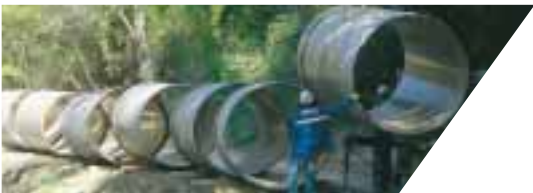
Pipe laying in south-eastern France.
