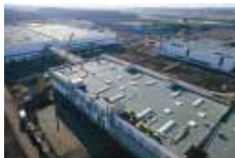
The MCC plant in Hambach.
