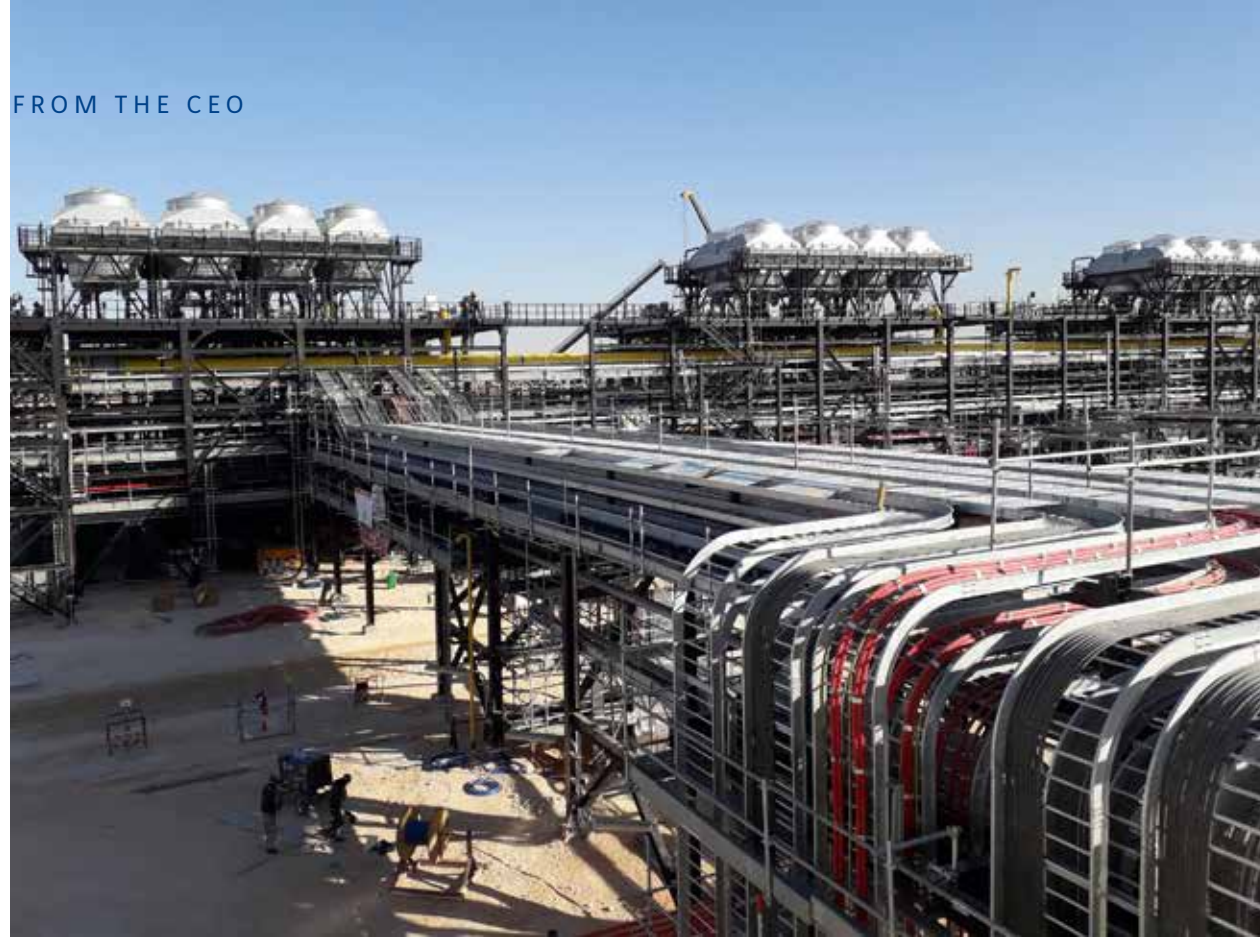
► Construction of a GOSP on the Upside North site in Algeria
