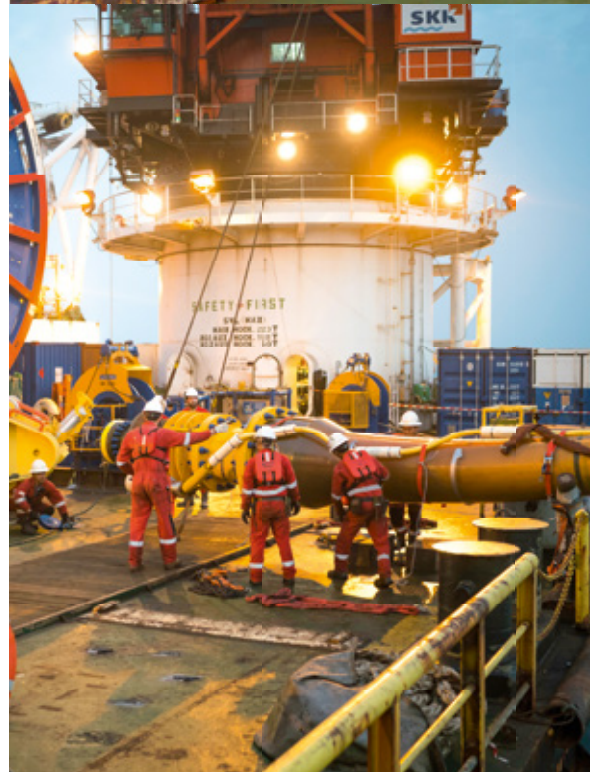
Connecting the riser to the plug
