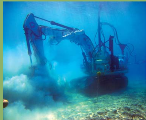
Abyss remotely-controlled submarine excavator, developed by Geocan and used in 2016 on the Escondida Water Supply Project in Chile.
