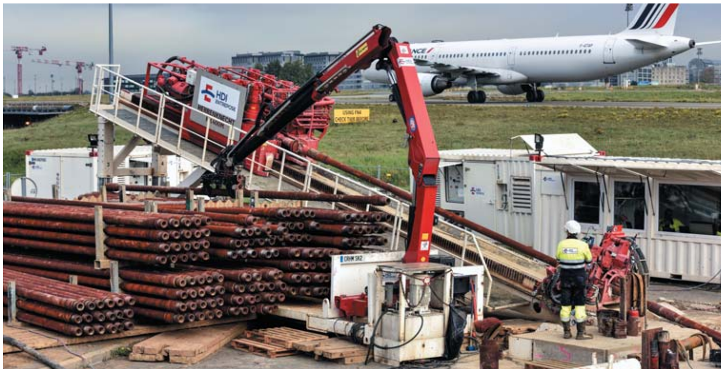
Horizontal directional drilling under the runways at Paris – Charles-de-Gaulle airport, France.
