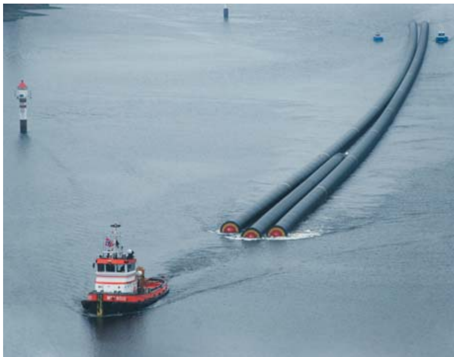
Towing HDPE pipes. Outfall project, Morocco.
