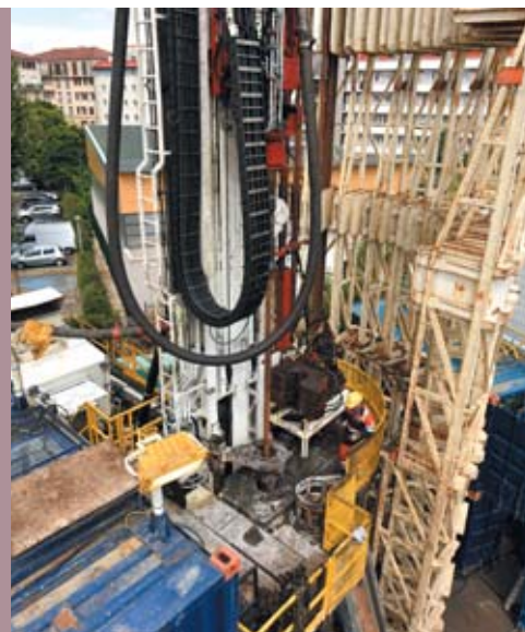
Creating geothermal wells in an urban environment, Chevilly-Larue, France.
