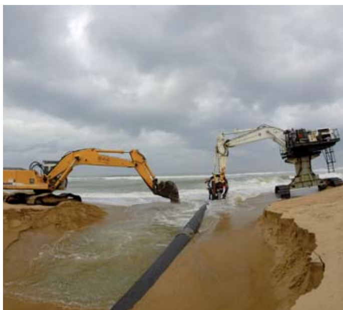
Trenching operation in Benin.
