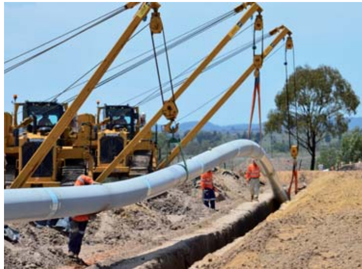
Installation of pipeline for QGC in Australia.
