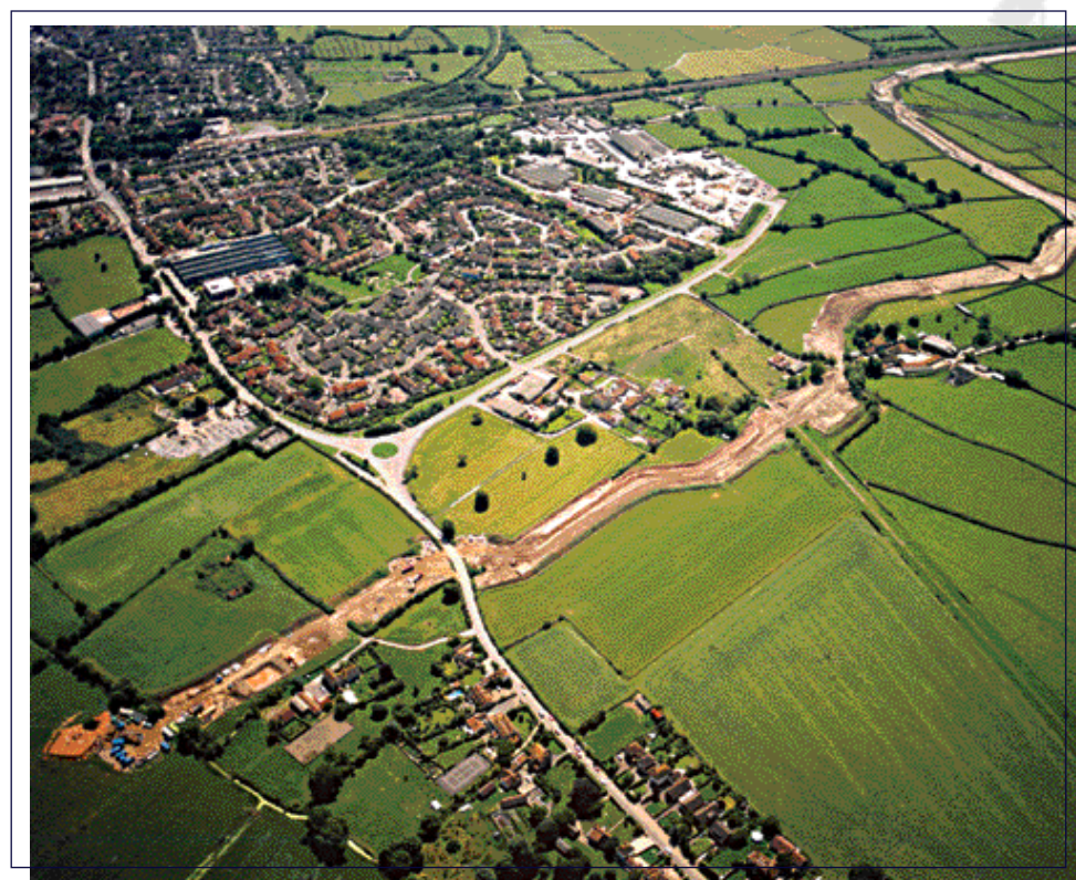
Pose de pipelines 48"-ROYAUME UNI / 48" pipelines installation-UNITED KINGDOM
