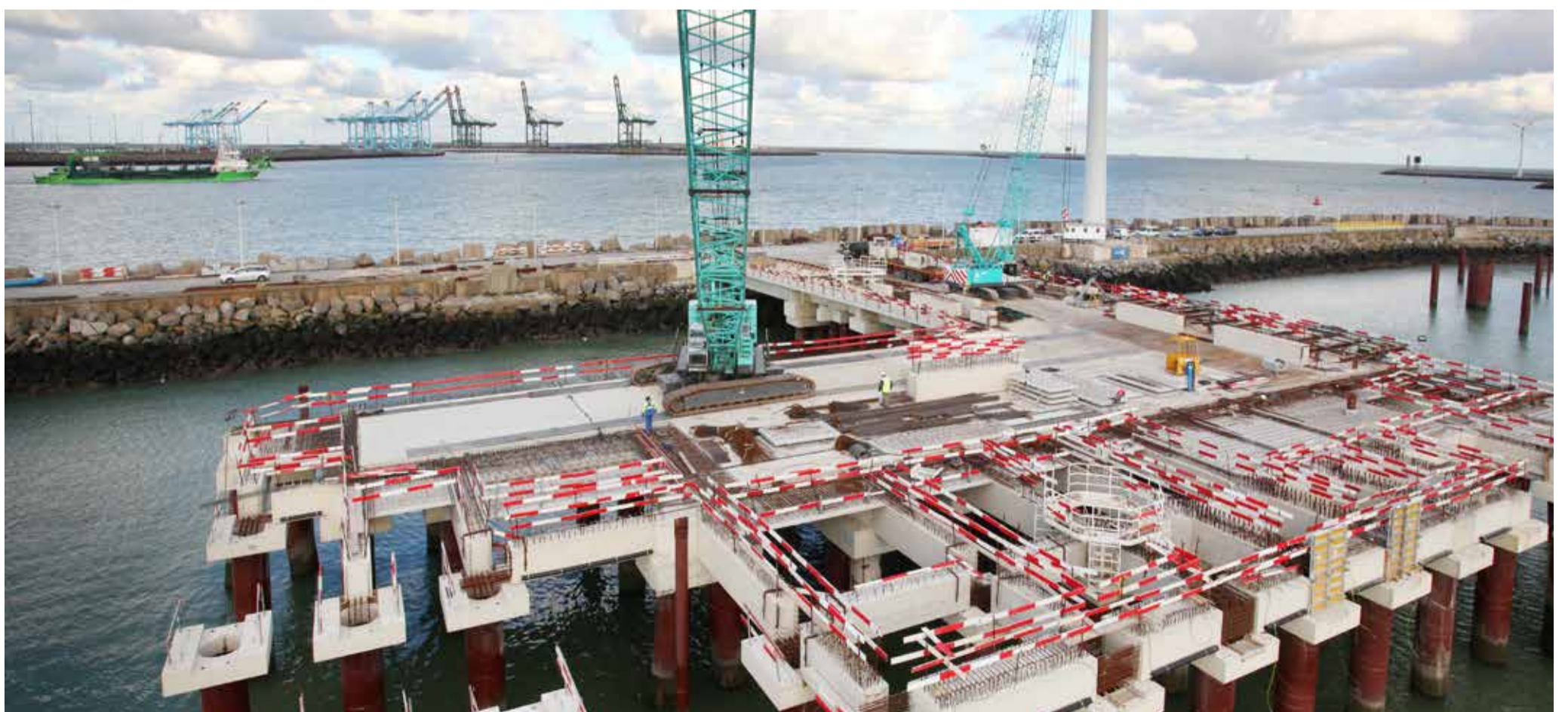
▲ Construction of a jetty for Fluxys - Zeebrugge
