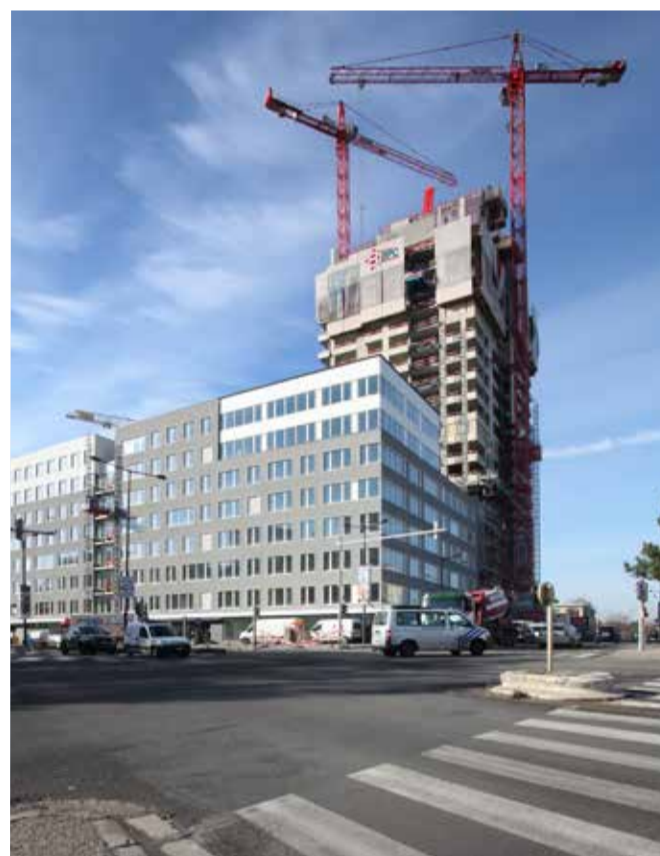
▲ Up-Site, the tallest residential block in Brussels
