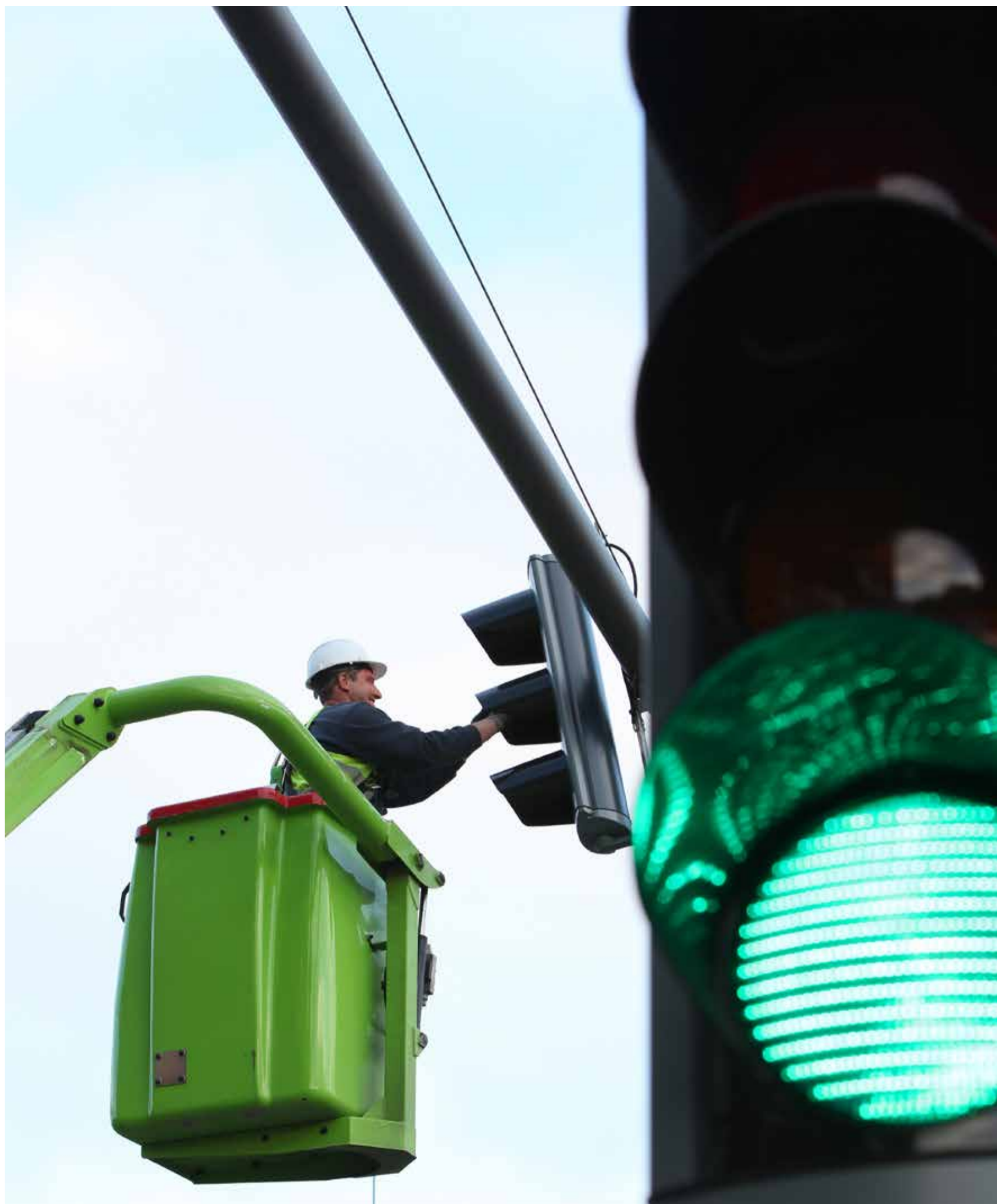
▲ Installing public lighting - Mons
