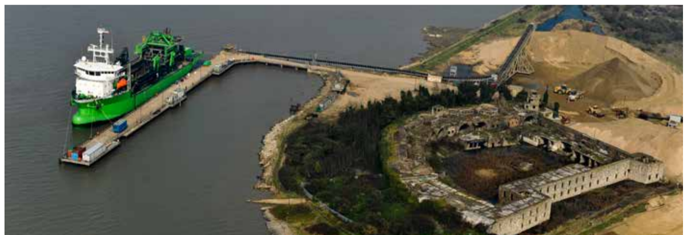
▲ Gravel trailer Victor Horta - London Gateway project (UK)
