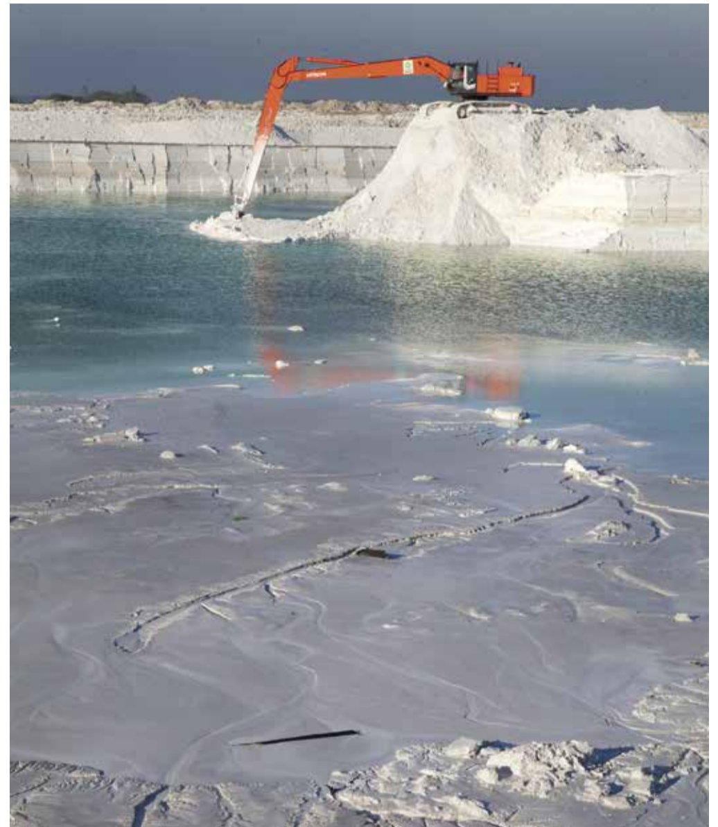
▲ Redevelopment of the Terranova site - Ghent
