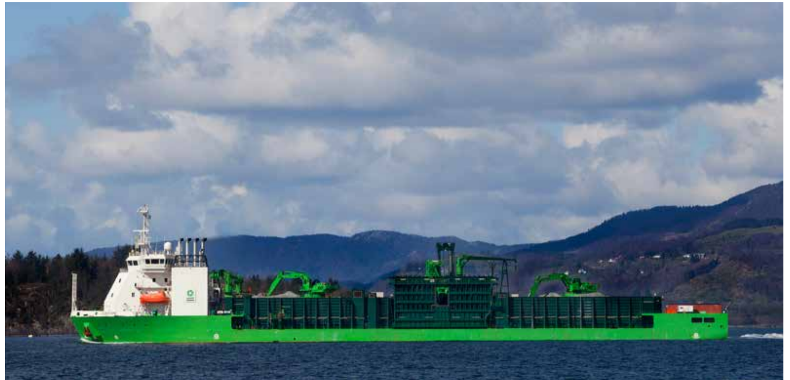
▲ Fallpipe vessel Flintstone - Norway
