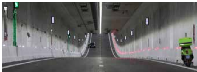
▲ Coentunnel - Amsterdam (NL)
