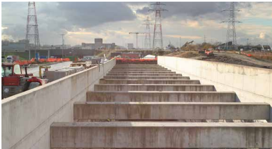
▲ Liefkenshoek railway tunnel - Antwerp
