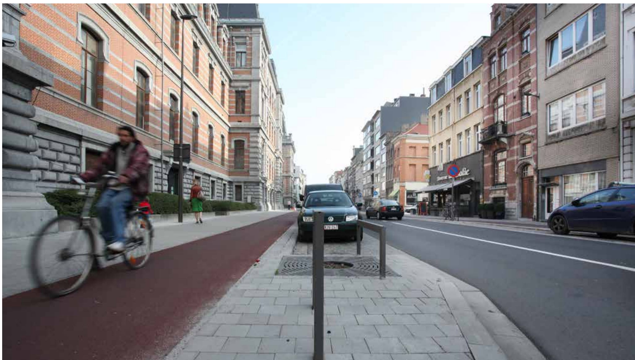
▲ Upgrading works of the Paleisstraat - Antwerp
