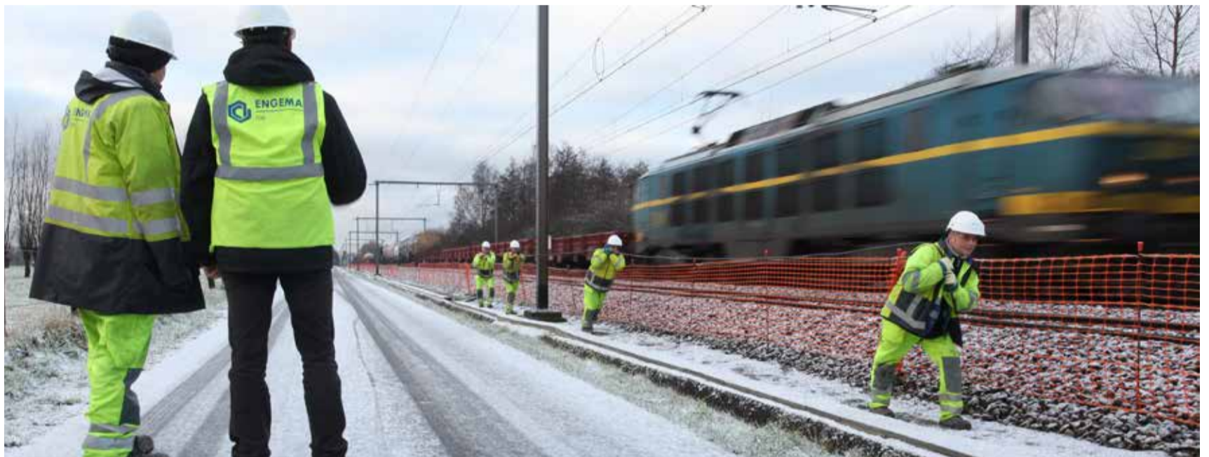
▲ Signalisation works - Lokeren
