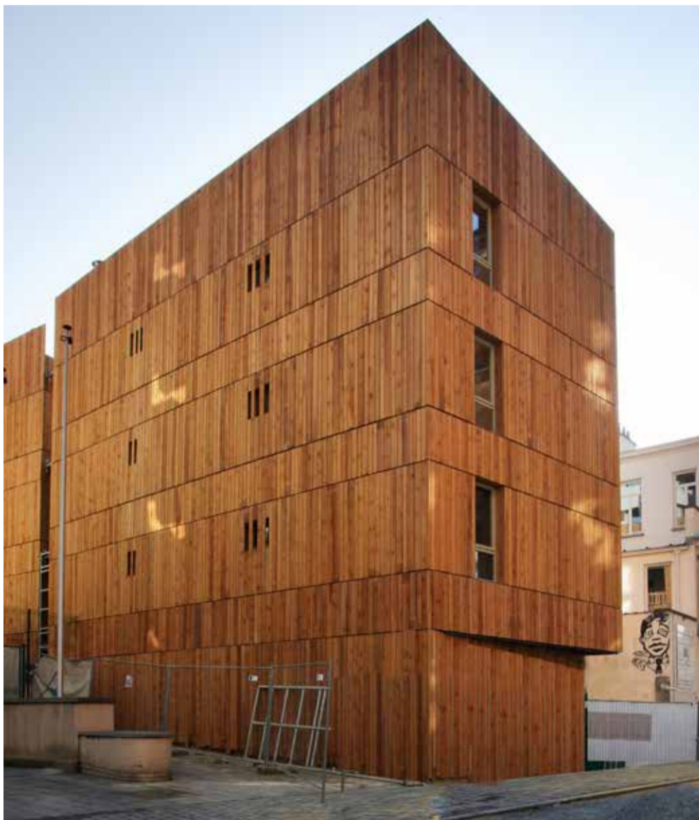
▲ Wood construction with high energy performance standards for the CPAS of Brussels
