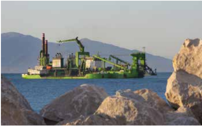
▲ Dredging works - Tanger (MAR)
