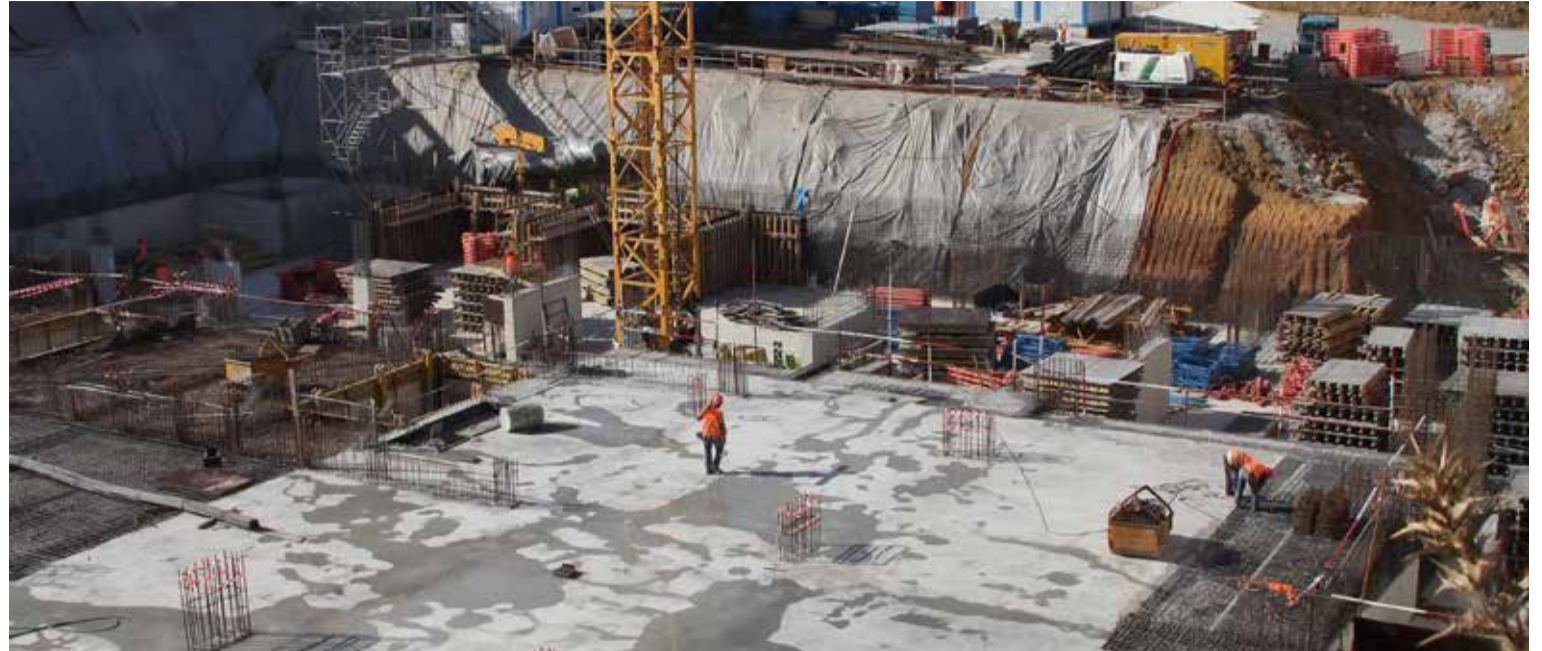
▲ Construction of the BNP Paribas head office in Algiers
