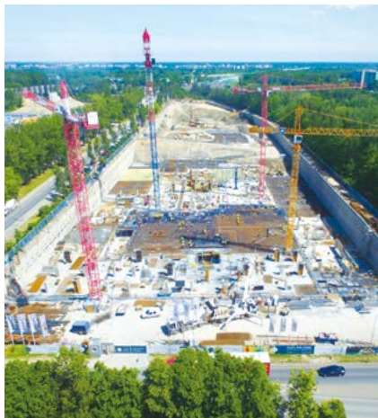
Mlociny gallery, Warsaw, Poland Soletanche Polska executed geotechnical works for the construction of the new shopping centre Mlociny, the largest one in Warsaw. We implemented an optimised solution comprising diaphragm walls over 1,000lm at an average depth of 16 metres, nearly 900 ground anchors and over 2,300 micropiles. The first clients came into the shopping mall May 23, 2019. #fostergrowth
