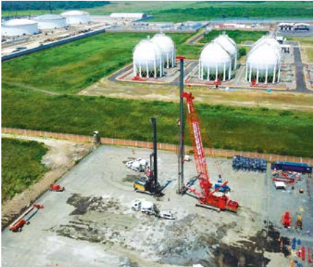
Controlled Modulus Columns & Vertical drains In Mexico, as part of the construction of an oil terminal in the port of Tuxpan in the state of Veracruz, Menard has supplied and installed 55,000 vertical drains and 5,500 Controlled Modulus Columns, the deepest ever built in Mexico. Once completed, the infrastructure will accommodate 10 fuel tanks. #fostergrowth #accesspower
