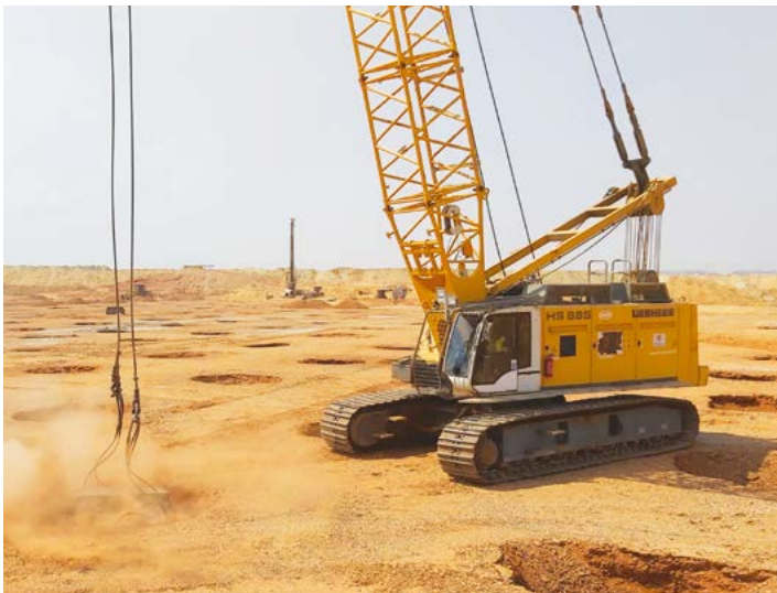
Dynamic Compaction Dynamic compaction of 80,000 square metres of soil: such is the challenge that Menard has set out to address in Egypt to stabilise and densify the soil on the site earmarked for the construction of the Celia complex, which will form part of the new administrative capital east of Cairo. #fostergrowth #makingyourdayeasier
