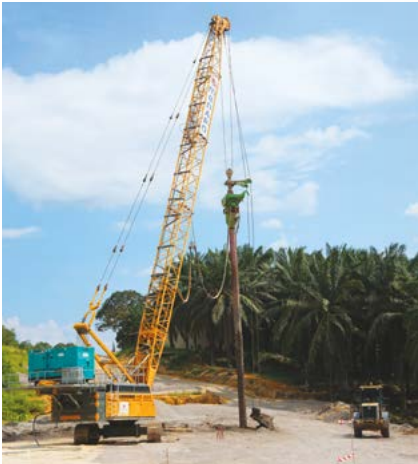
Stone columns One metre in diameter, 230,000 linear metres in total, these are the dimensions of the stone columns supplied and installed by Menard in Malaysia as part of the construction of a new electrified railway line. With planned works taking place without any rail traffic downtime, the new infrastructure is expected to save passengers 2.5 hours on their journey between Gemas and Johor Bahru. #makingyourdayeasier
