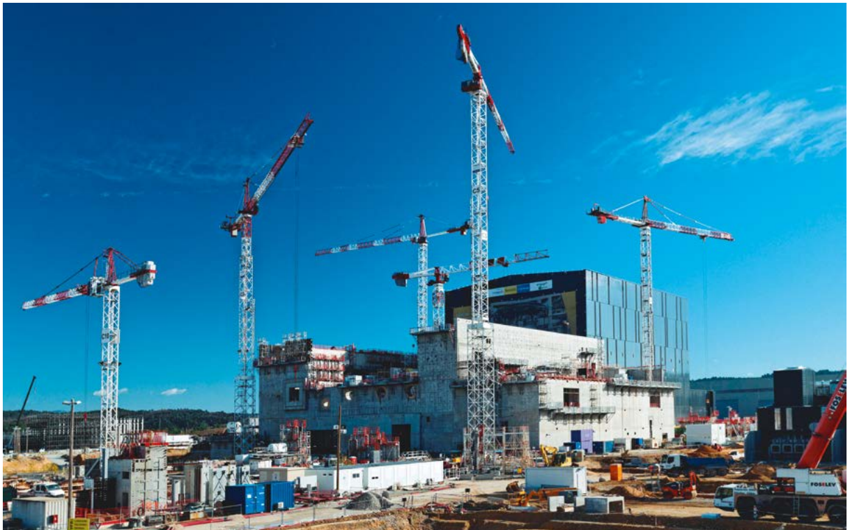
Construction of the experimental ITER nuclear fusion reactor, one of the world’s largest nuclear research programmes. VINCI Construction leads a consortium working on the project.
