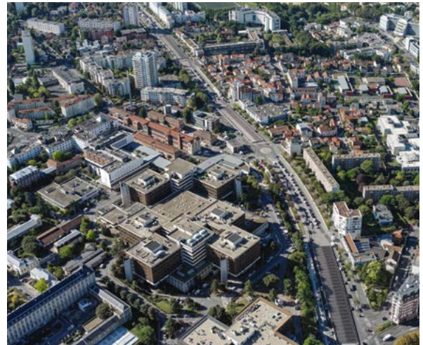
VINCI Construction won the first civil engineering works package on the Line 14 South extension that will connect Paris with Orly Airport.
