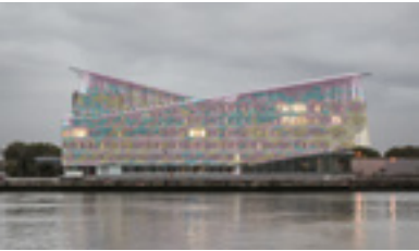
The 108 in Rouen, France: built in accordance with an HQE® Bâtiments Tertiaires high environmental quality programme, the new Métropole Rouen Normandie headquarters aims for exemplary thermal and energy efficiency.
