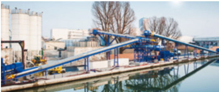
Conveyor belt installed to remove rubble from the metro Line 12 project in Paris by barge via the Saint Denis canal.
