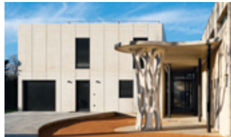
The first 3D printed column in a school courtyard in Aix en Provence, France.
