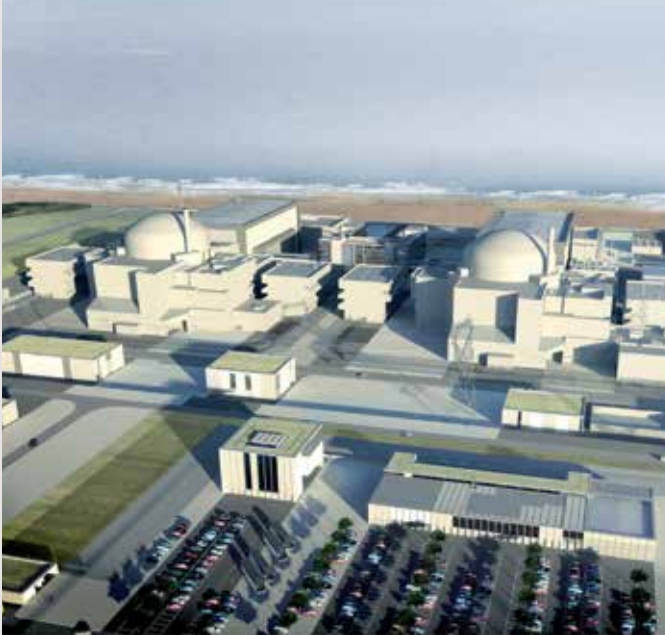
Hinkley Point, United Kingdom: construction of two EPR nuclear reactors.
