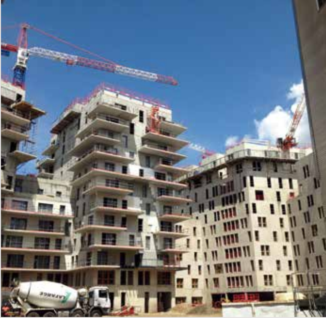
Girondins development zone in Lyon, France: construction of 837 housing units.
