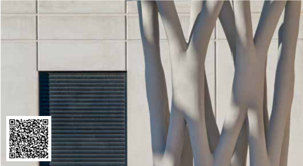
3D printing is used to produce complex concrete shapes such as this 4-metre pillar supporting the covered courtyard at a middle school in Aix en Provence (France).
