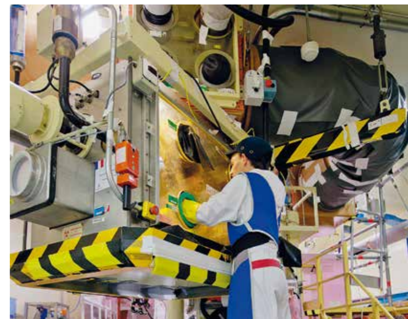
CADARACHE // FRANCE Decommissioning of a glove box
