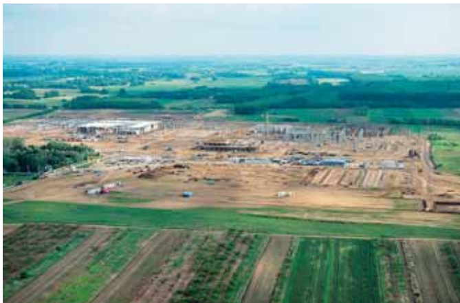
Lego plant, Nyiregyh za, Hungary HBM (Soletanche Bachy) built the foundations of the new Lego plant in eastern Hungary, installing more than 50 km of reinforced concrete piles and 7,000 cu. metres of pile heads.
