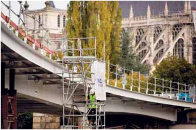
Paris Bridge, Beauvais, France ^ Sogea Picardie (VINCI Construction France) deconstructed and reconstructed the 120 metre long curved structure built in 1949, installing a new metal deck.
