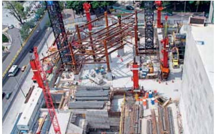
BBVA Bancomer tower, Mexico City, Mexico Soletanche Bachy's Mexican subsidiary Cimesa built 24,000 sq. metres of perimeter diaphragm walls (width: 1 metre), barrettes (up to 50 metres depth and 1 metre width) and 156 circular piles (1.40 metre diameter, 40 metre depth) for the foundations of this tower.
