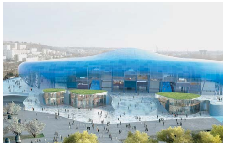
The Grand Stade in Le Havre, built by VINCI Construction France, will be one of France's very first positive energy stadiums thanks in particular to 1,500 sq. metres of photovoltaic cells installed on its roof.
