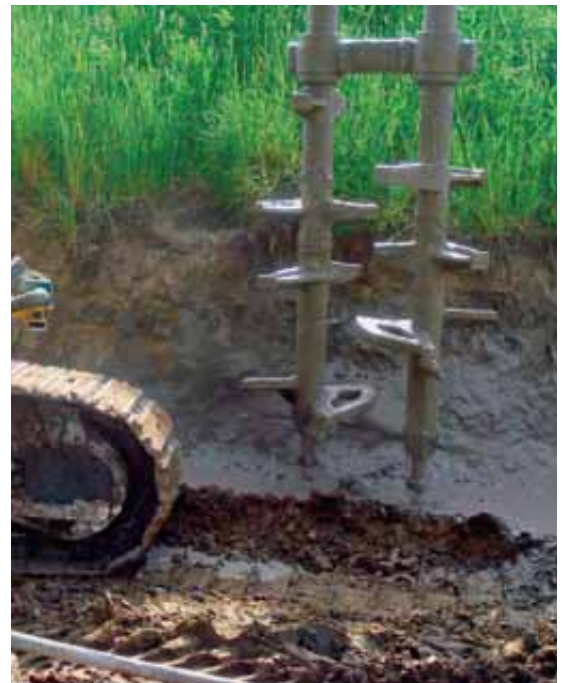
ENVIRONMENT. Menard used the soil mixing technique, carried out with a twin auger, to remediate a chlorine-contaminated brownfield site in southeastern France.
