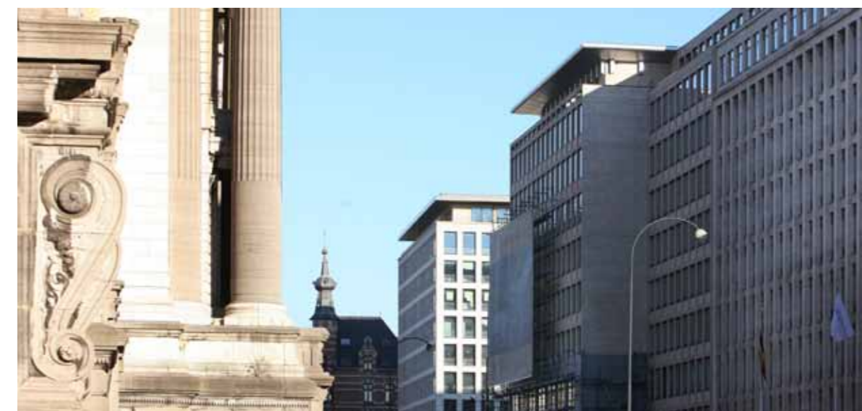
Renovation of the 'Justice' building – Brussels (BE)
