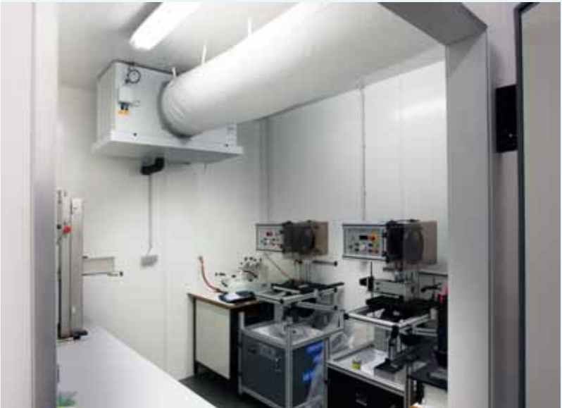
Installation of cooling equipment - Brussels (BE)
