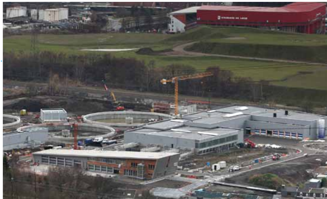
Installation of the electromechanical equipment – Sclessin (BE)
