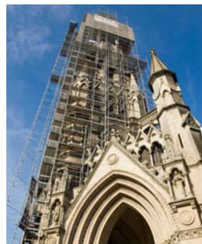
Repairing the reinforced concrete bell tower of the Sacré Cœur church in Lille.
