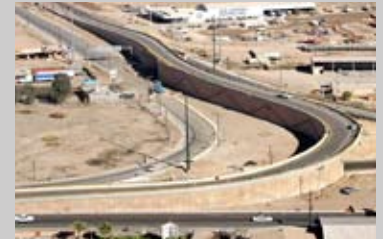
Construction of 70,000 sq. metres of reinforced earth walls by Terre Armée on 16 engineering structures in Mexico.
