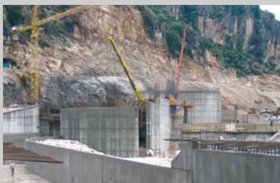
Hydroplus, a subsidiary specialising in raising the height of dams, is installing nine fusegates on the Dafnozouara dam in Greece.
