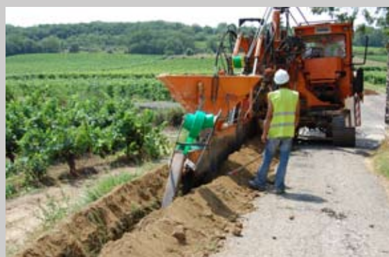
Laying optical fibre cable to roll out a broadband telecom network for the Hérault department, France.
