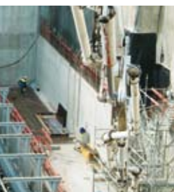
3 United States: construction of two 6.1 and 3.6 km tunnels (the external diameter of the tunnelling machine is 5.3 metres) to supply the new Brightwater wastewater treatment plant, north of Seattle.
