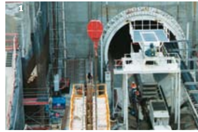
1 Marseille Metro: digging a nearly 2 km long, 9.79 m diameter tunnel. The project also includes the building of the la Fourragère station and two ventilation shafts.
