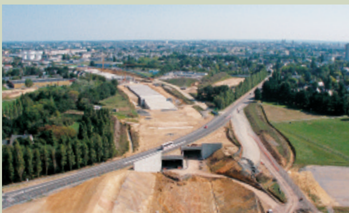
A consortium comprising a majority of VINCI Construction companies is building the northern Angers bypass on the A11 motorway for Cofiroute. The project includes 5 interchanges, 16 standard structures, 1,700 metres of cut and cover and a 530 metre viaduct over the Maine River.
