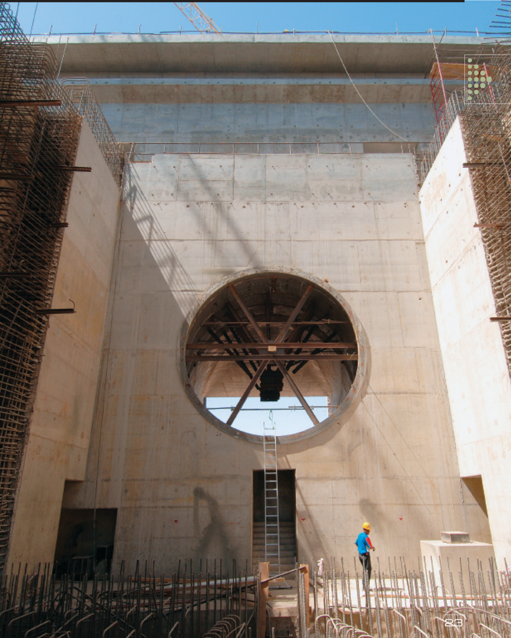
The Naga Hammadi dam, built by VINCI Construction Grands Projets in Egypt, will be commissioned in 2008 following 72 months of work.
