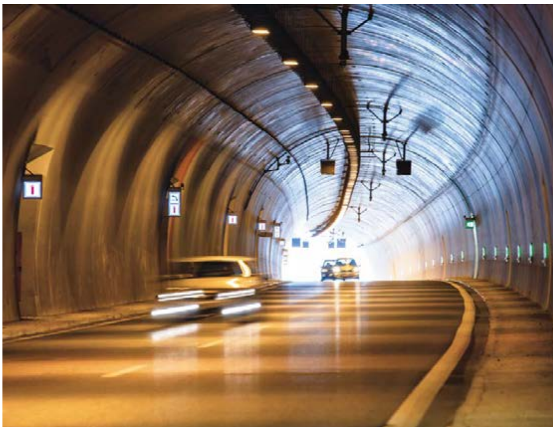
LED lighting in tunnels improves driver comfort in Greece's Athens-Patras highway.
