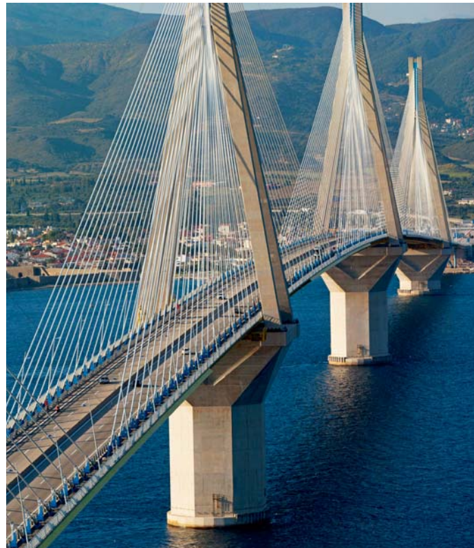
The Charilaos-Trikoupis bridge, built and operated by VINCI, marked its 10 th year of operation in 2014.
