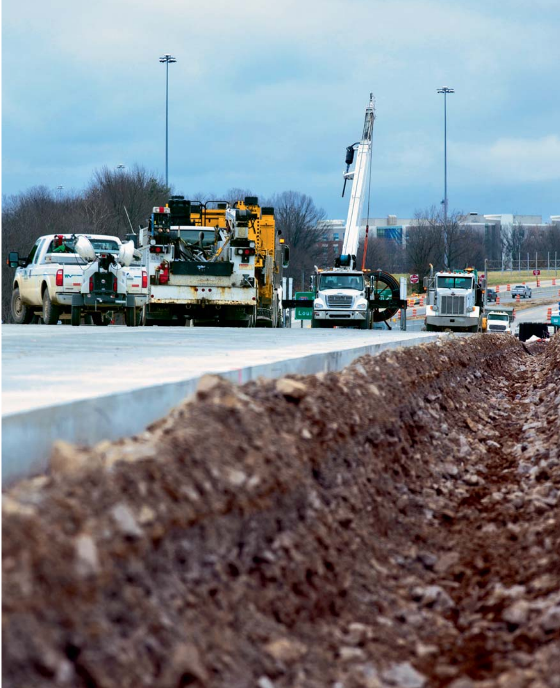
Construction of the East End Crossing should be completed in fall 2016, just four years after award of the contract.
