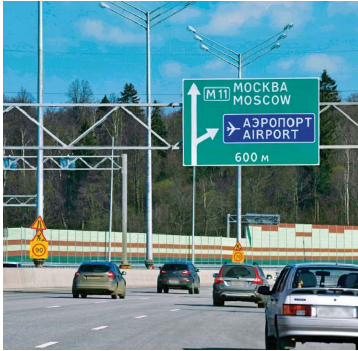
Connecting the Moscow beltway with Sheremetyevo International Airport, the new infrastructure thins the traffic in the fully saturated area.
