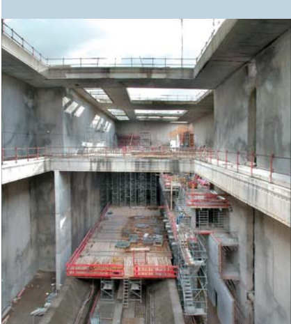
A13 interchange Construction of the bottom slab extension of the tunnel at the A13 interchange
