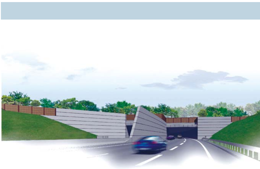
Entry to cut and cover on A11 Angers
