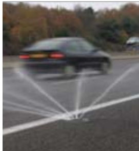
> Salt water sprinklers on the A10
