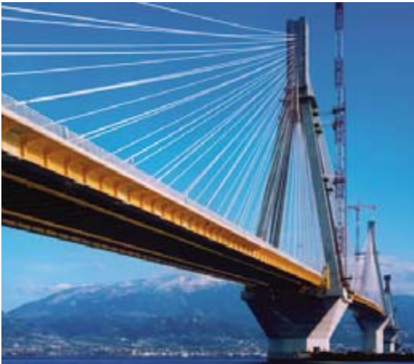
&gt; Rion-Antirion Bridge
