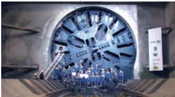
> The tunnel boring machine emerges on 14 October 2003
