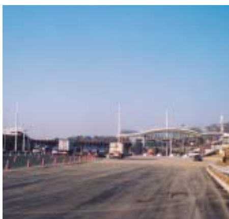
Extension of La Négresse toll station – A63
