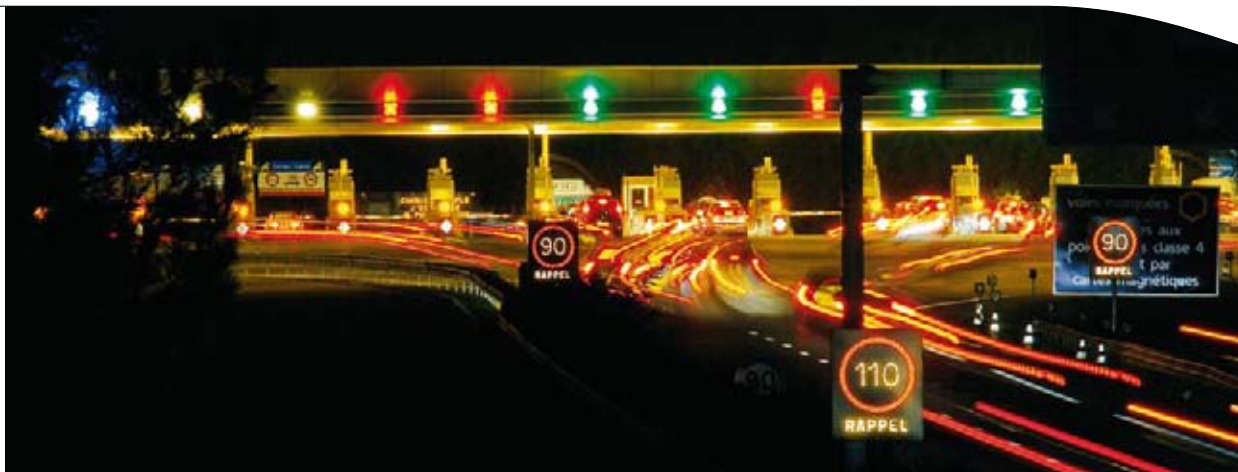
A major programme commitment to optimise the existing network.
