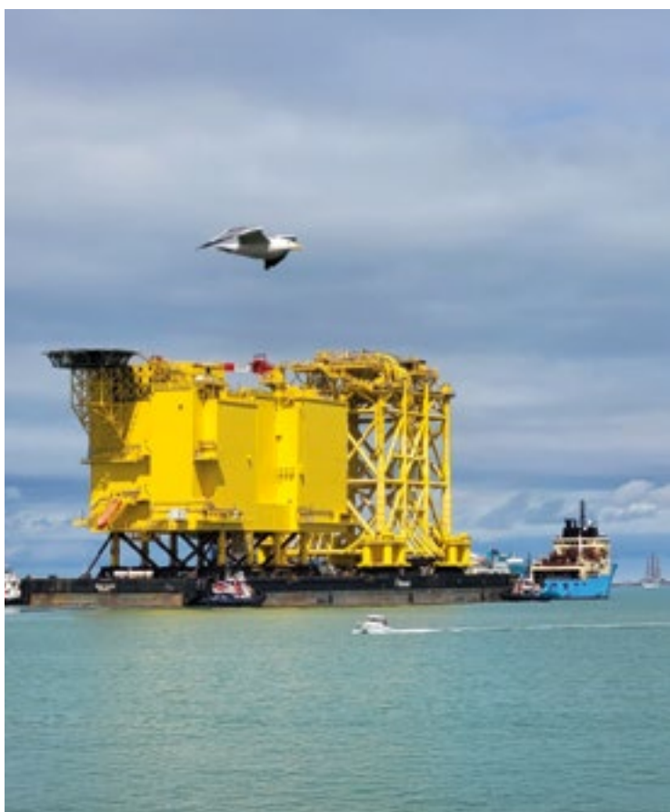
Dragados Offshore transferred and installed the topsides and jacket for the BorWin5 HVDC converter platform (900 MW), in the North Sea. Four other platforms are under construction in Spain.
