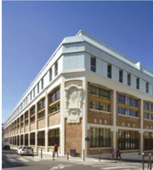
In the 13th arrondissement of Paris, the Télécom Paris building was restructured into three parallel lots. The three sites presented common issues, such as a narrow footprint and difficulties related to working in a dense urban area.
