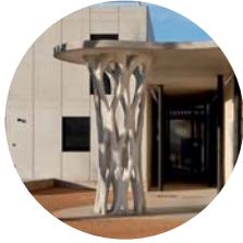
VINCI CONSTRUCTION IS WORKING WITH XTREEE, A STARTUP, TO DEVELOP CONCRETE 3D PRINTING.
