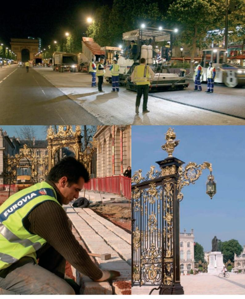
**Top.** The low production and application temperature of warm mix with Aspha-Min<sup>®</sup> reduces emissions of greenhouse gases. On the Champs-Elysées in Paris, the process was employed for the first time during the events staged to support Paris's bid for the 2012 Olympic Games.
