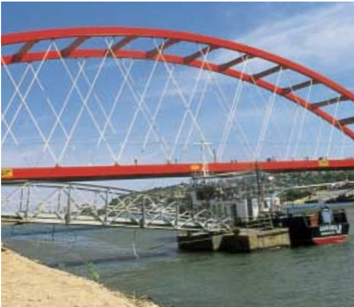
To install the roadway of the Cernavoda metal bridge in Romania, Freyssinet rotated it on a barge, thus reducing downtime to a minimum.
