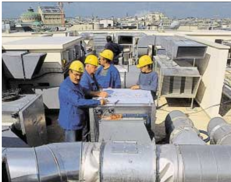
Installing air-conditioning and smoke evacuation systems on one of the buildings of the AXA insurance group in the 8th district of Paris.
