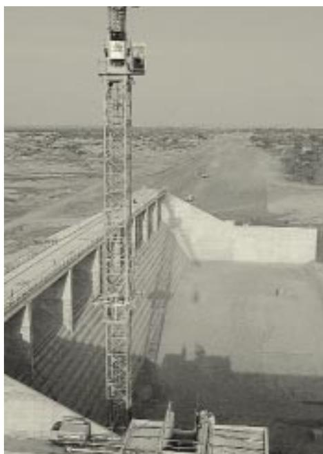
Sogea has a very tight deadline to complete the Ziga barrage in Burkina Faso. A main feature of the project is its use of a special type of compacted cast concrete. In all, 36,000 cu. metres of concrete will be used.
