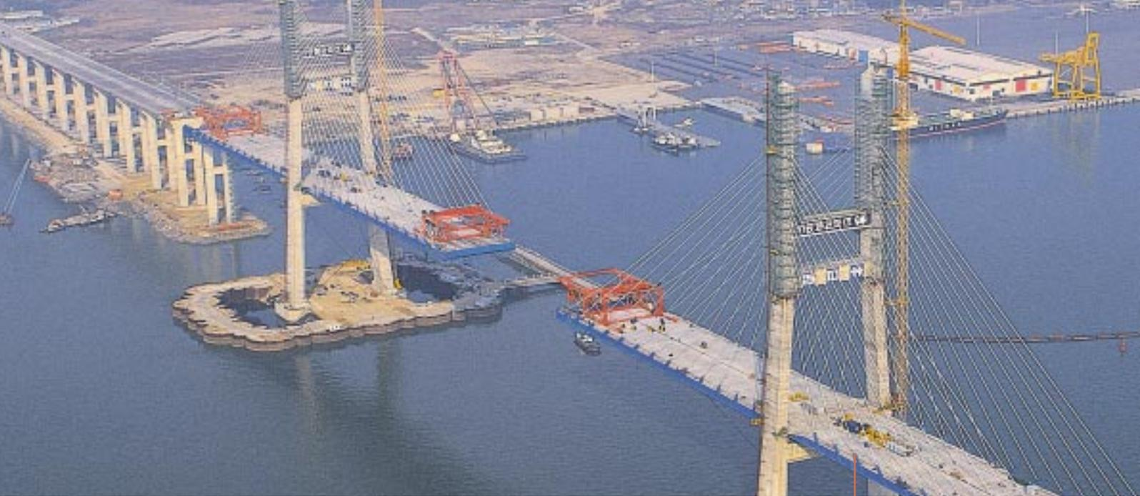
Freyssinet supplied the prestressing for pylons and stay cables on the Seohae bridge in Korea.
