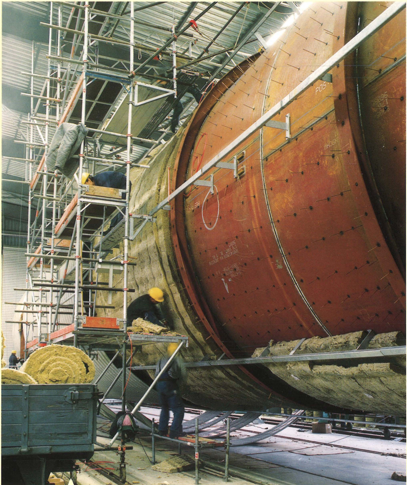
Laying of insulation inside the Jänschwalde power generation plant near Dresden.
