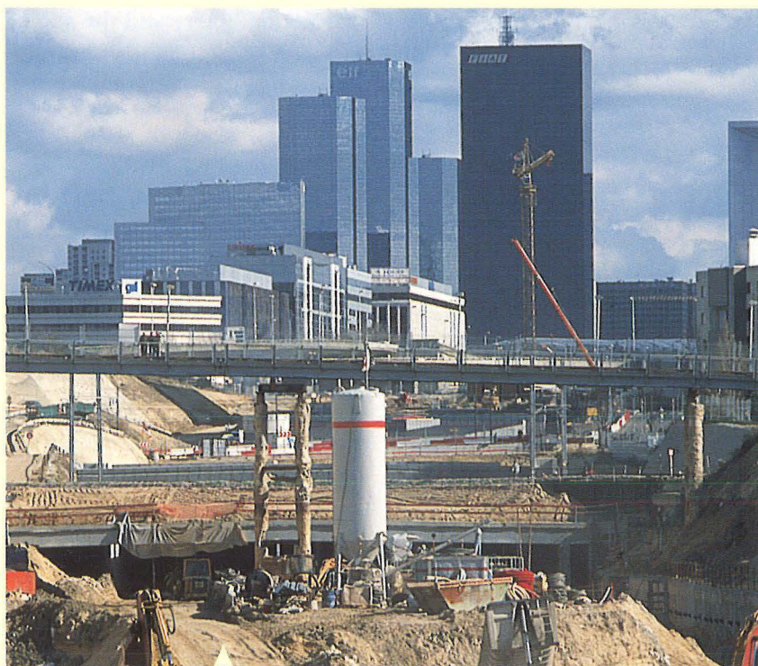
Sogea and its subsidiary TPI Ile-de-France, using the cut-and-cover method, are building the first section of the A14 motorway, which will link La Défense to the Normandy motorway at Orgeval.
